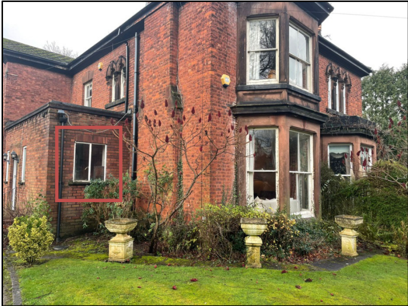
Existing steel window to be replaced
