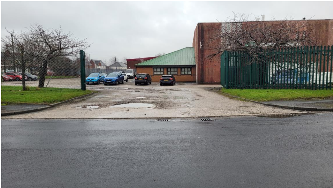
Photograph 4 – Existing access to main car park
