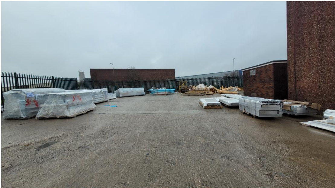
Photograph 2 – Existing hardstanding to rear of site
