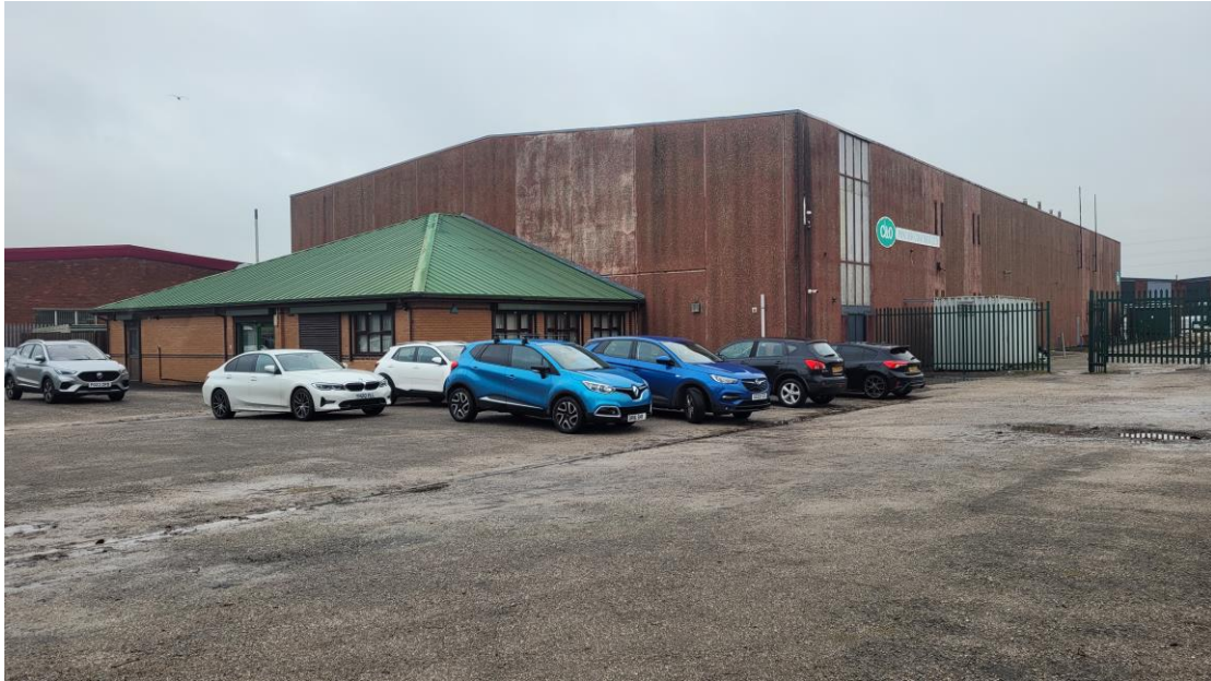
Photograph 1 – Front elevation & main car park
