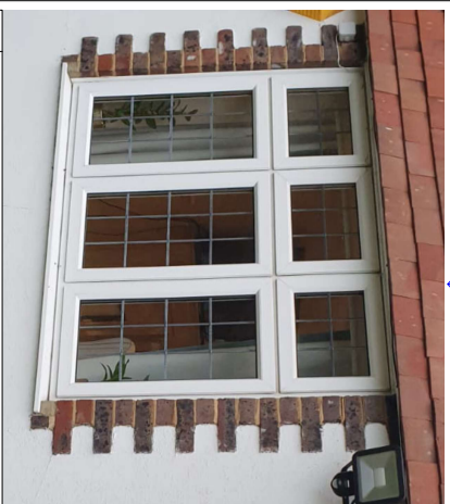
Existing windows: White UPVC flush framed double glazed windows with decorative stuck-on lead beads
