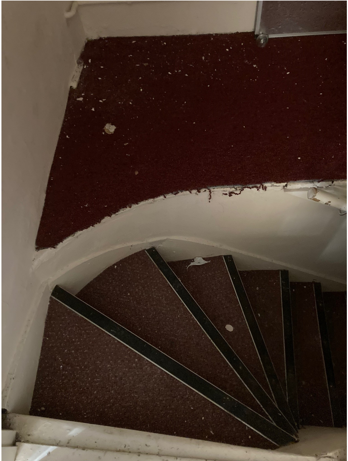
STAIR DOWN TO BASEMENT
