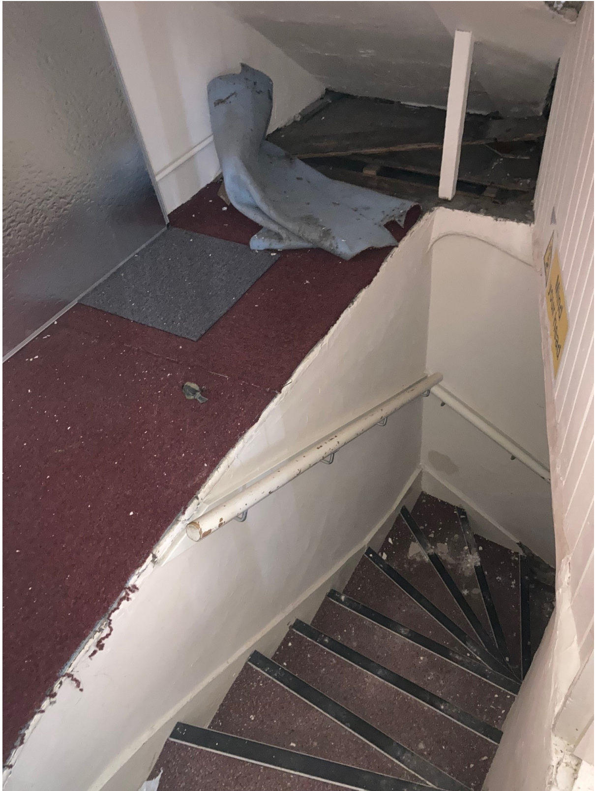
STAIR DOWN TO BASEMENT
