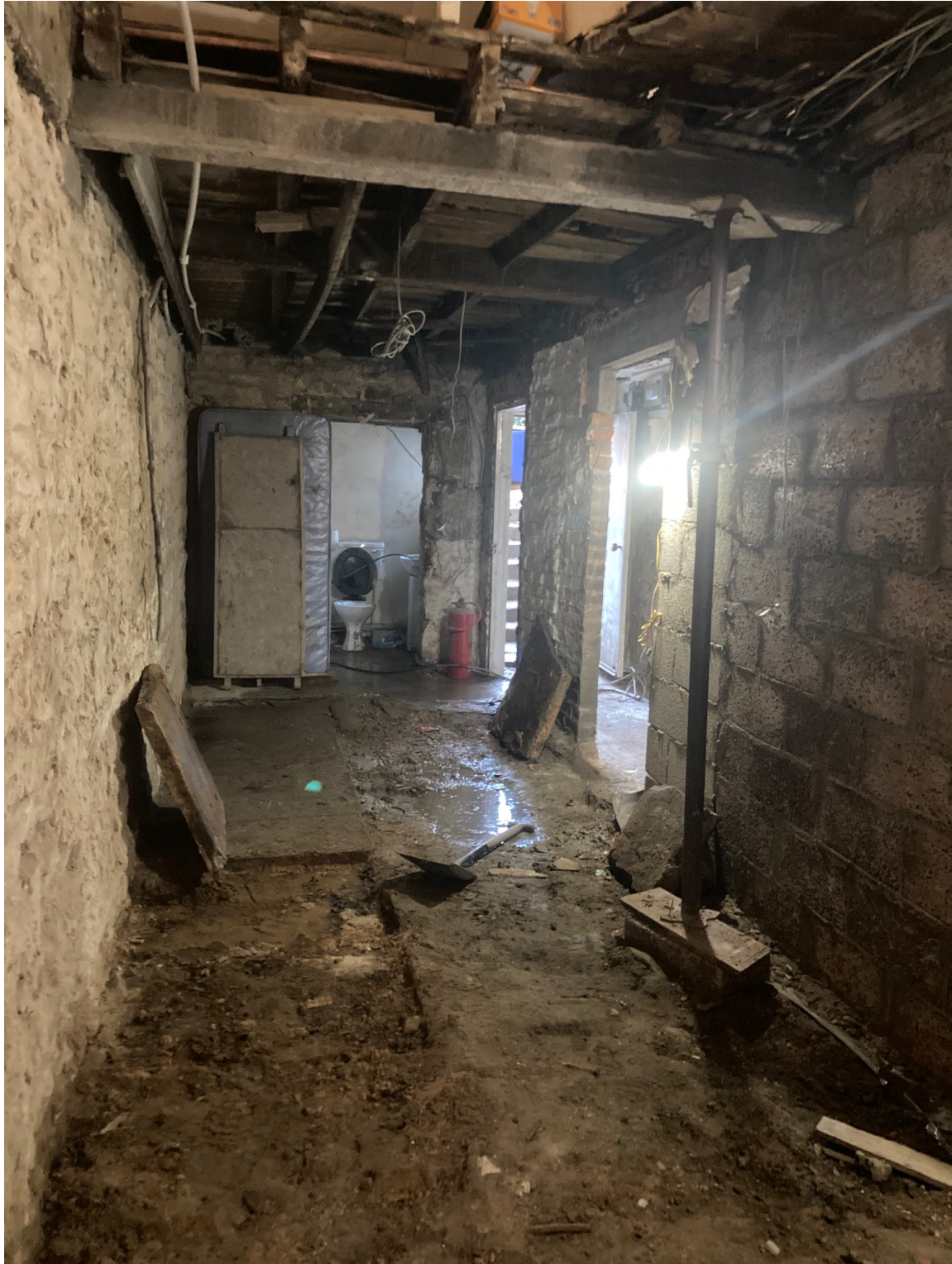
BASEMENT LOOKING TOWARDS EXISTING WC
