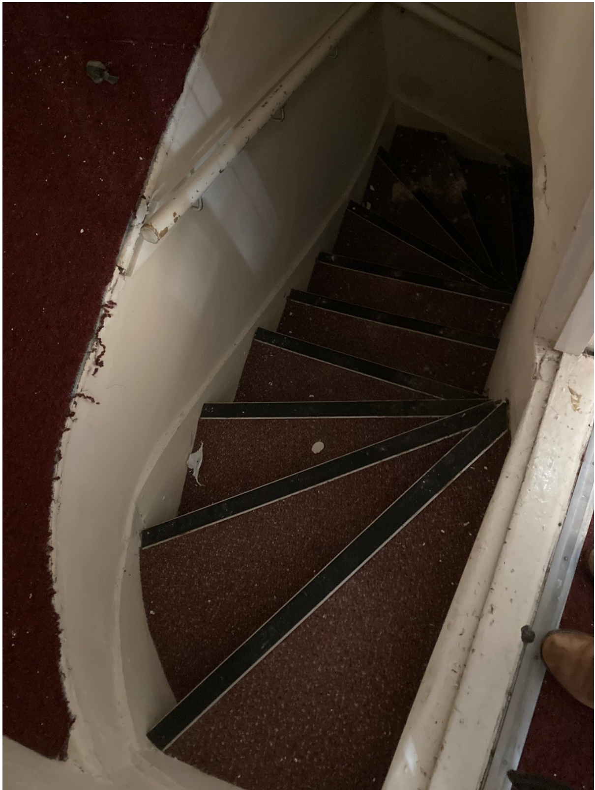
STAIR DOWN TO BASEMENT
