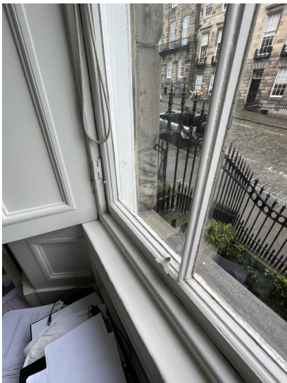
Ironmongery is non-existent in areas and requires to be installed. Gaps to window frame and sash are allowing draughts to enter property.
