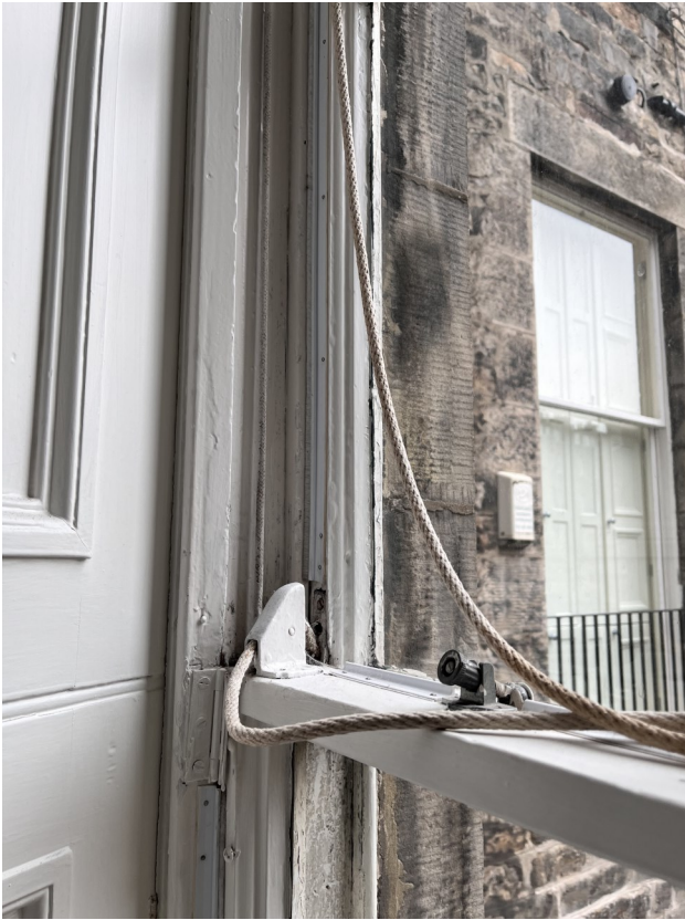
Defective rope cords do not allow for ease of opening for the user
