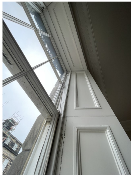
Ironmongery is non-existent in areas and requires to be installed. Gaps to window frame and sash are allowing draughts to enter property.
