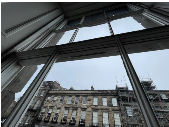
Ironmongery is non-existent in areas and requires to be installed. Gaps to window frame and sash are allowing draughts to enter property.
