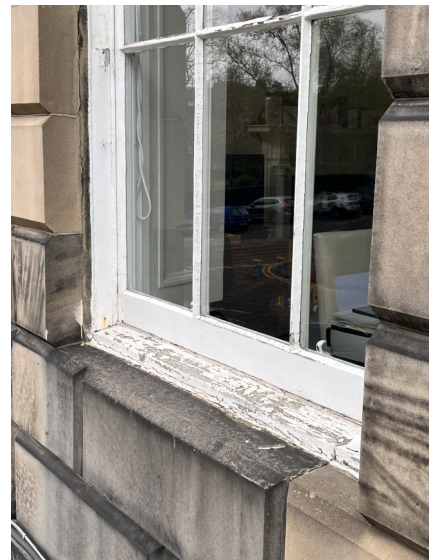
Defective cill requires to be replaced/ repaired.
