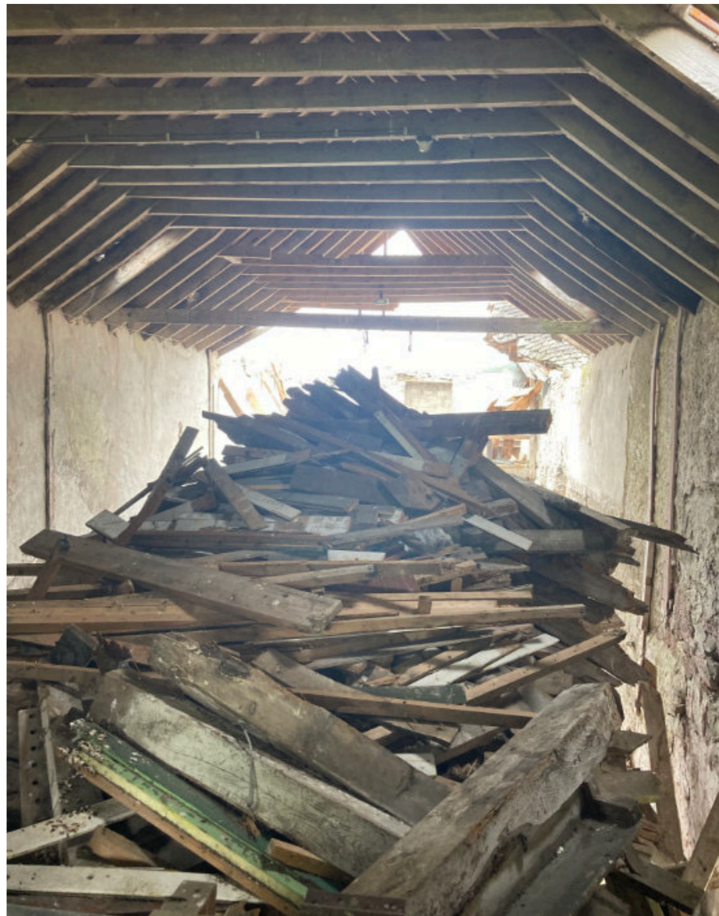
Interior of mill from West access, upper level, looking East.
