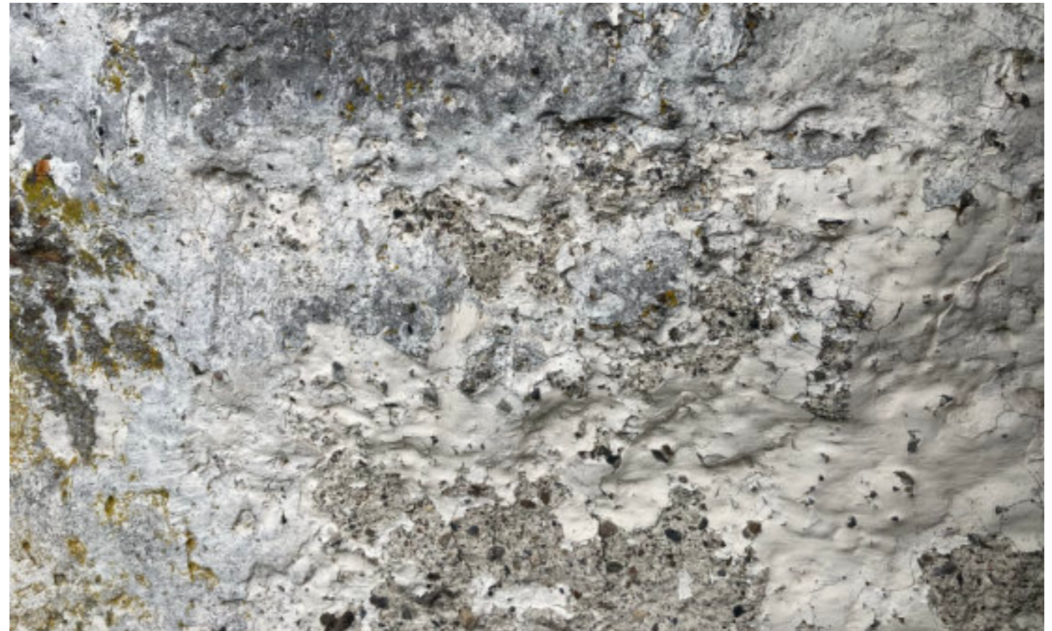
External elevation appears to have been lime rendered/limewashed historically
