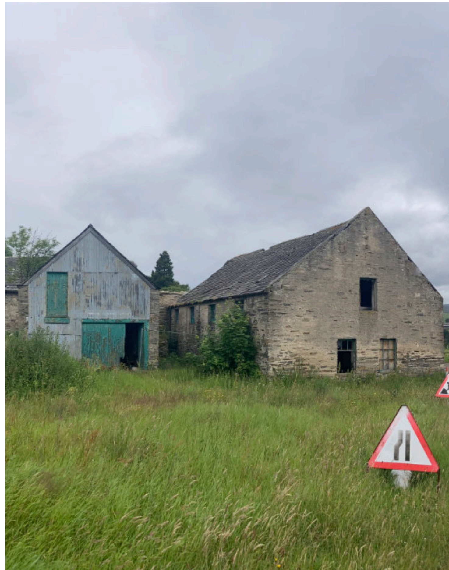
South gable of mill building
