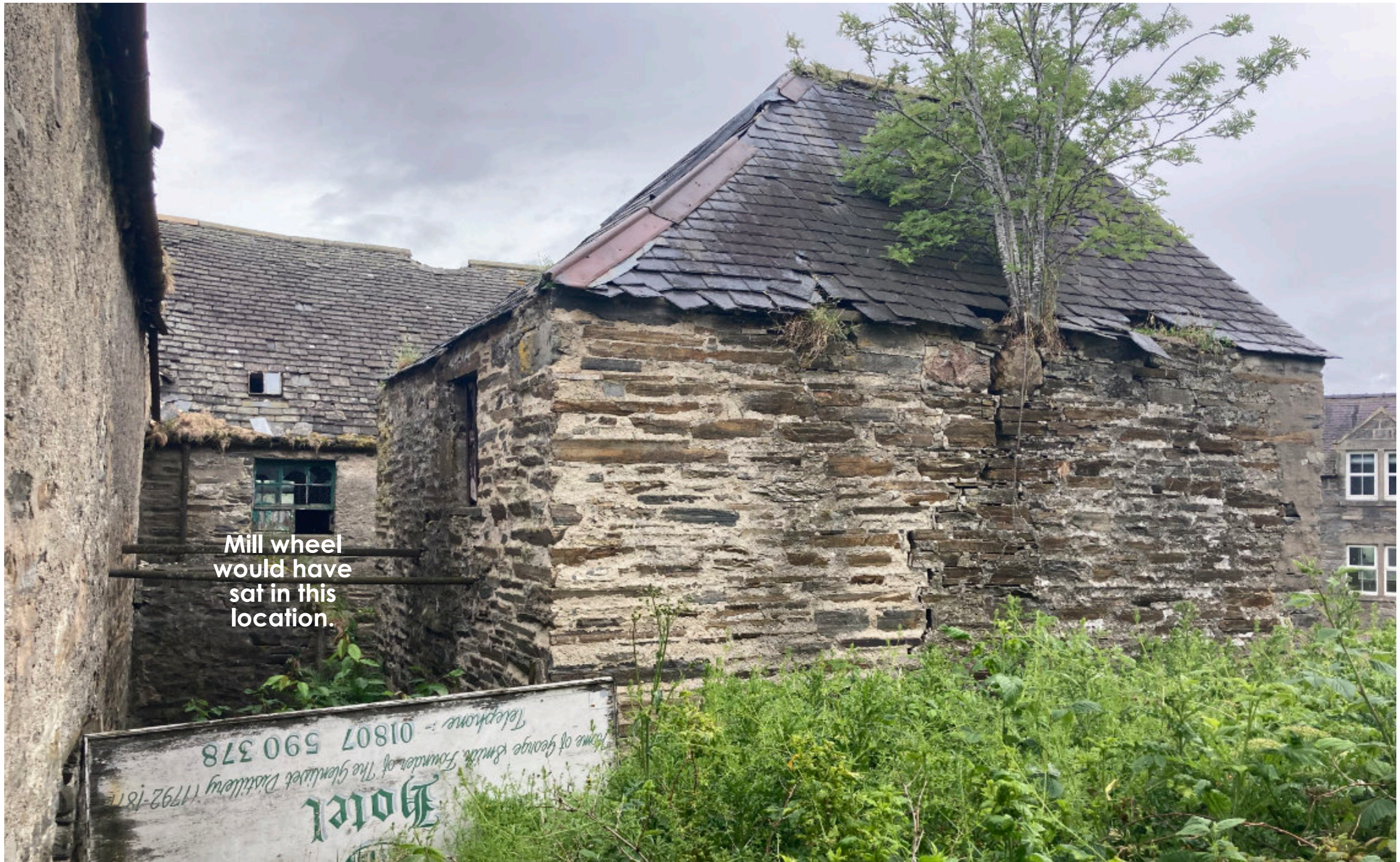
Area between mill and detached structure. - West Elevations - Note level of damage to external wall at right hand of image
