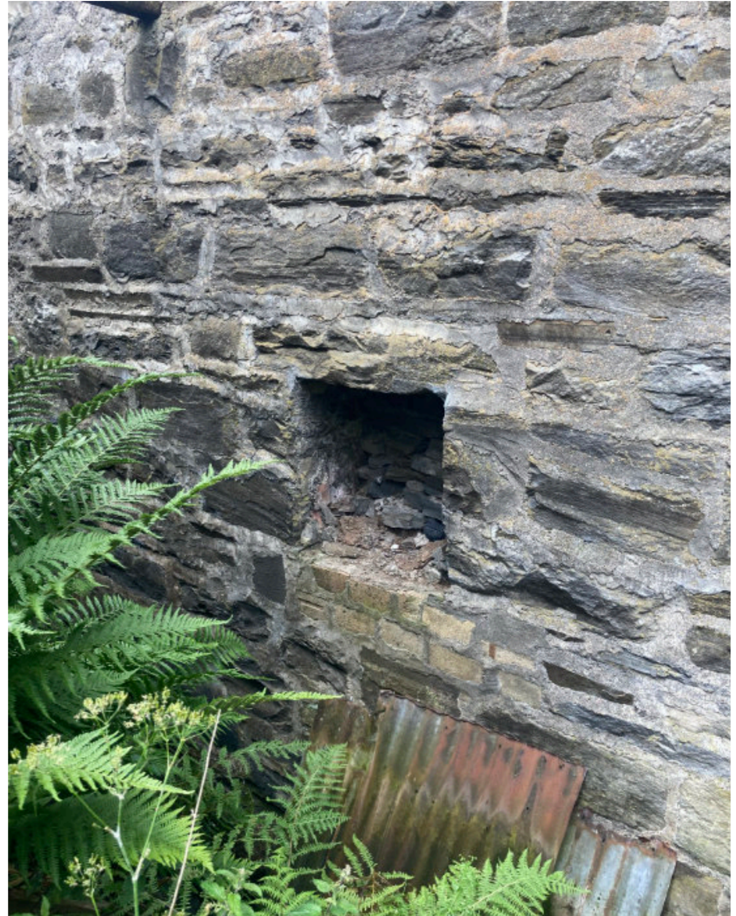
Historic mill wheel opening
