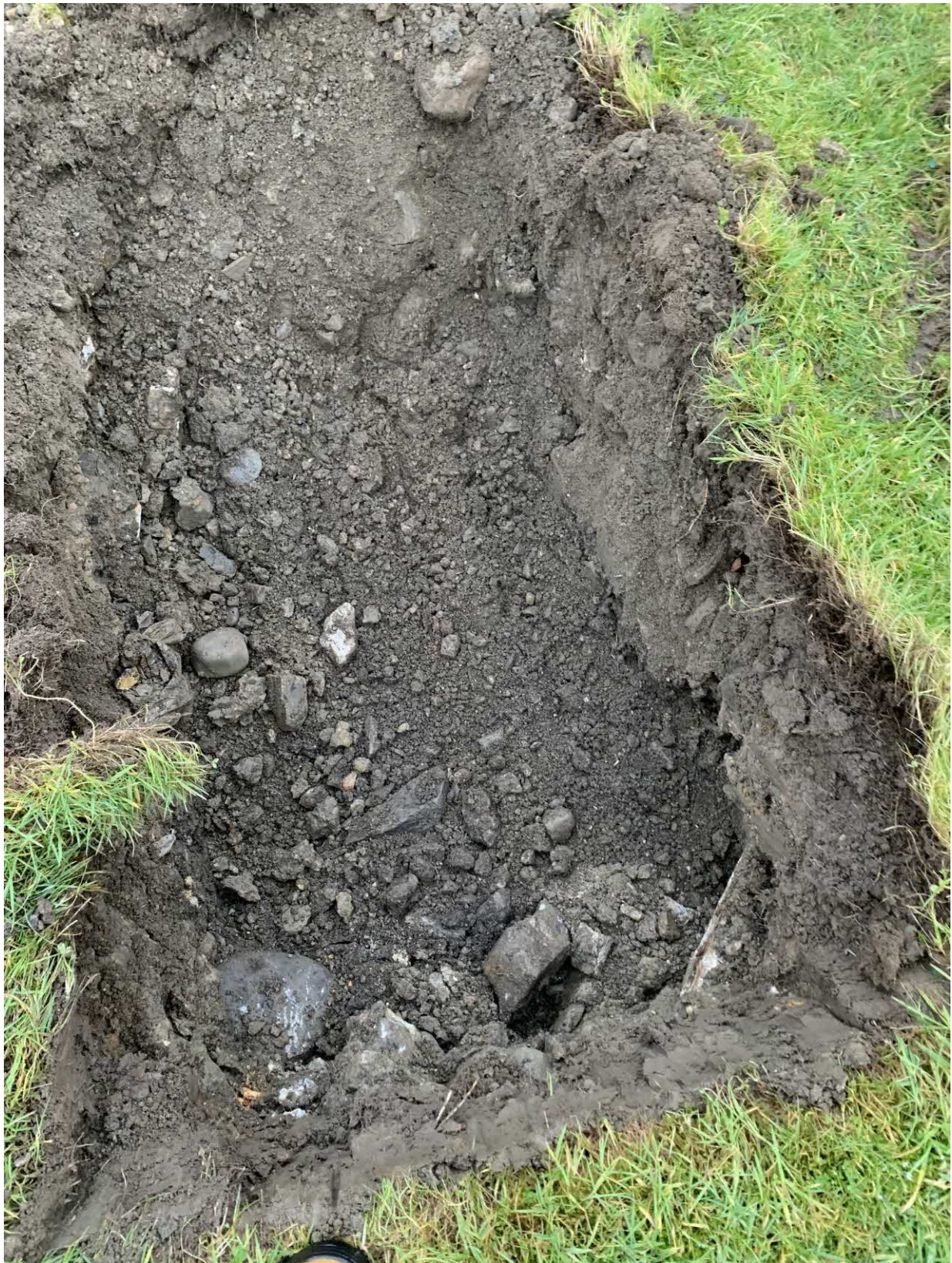
Photo of Trial Pit 1 (Trial Pit 2 is Identical)
