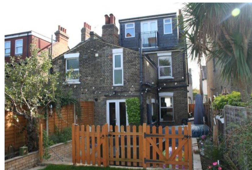
Rear view facing no.17
