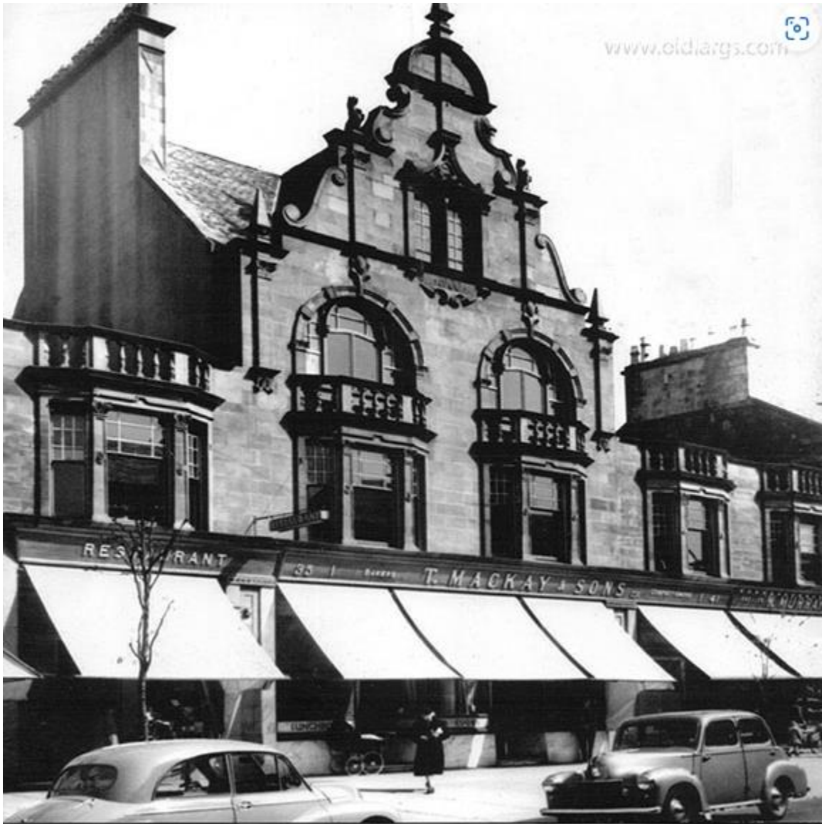
Street View 1950's Showing First Floor Stone Balustrades And Pinnacles Still In Position & Considerable Ground Level Glazing With Retractable Shades.
