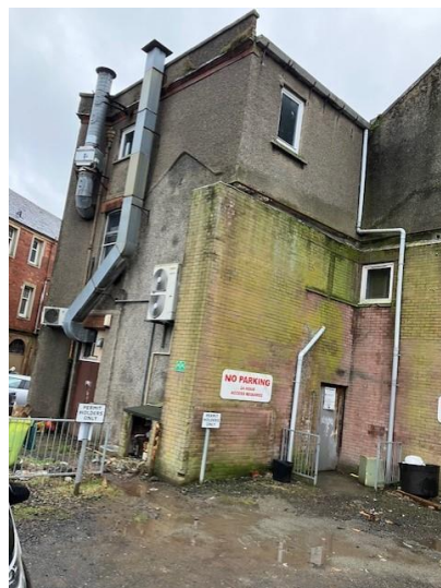
Rear Elevation Showing Myriad Of Finishes & Physical Interventions
