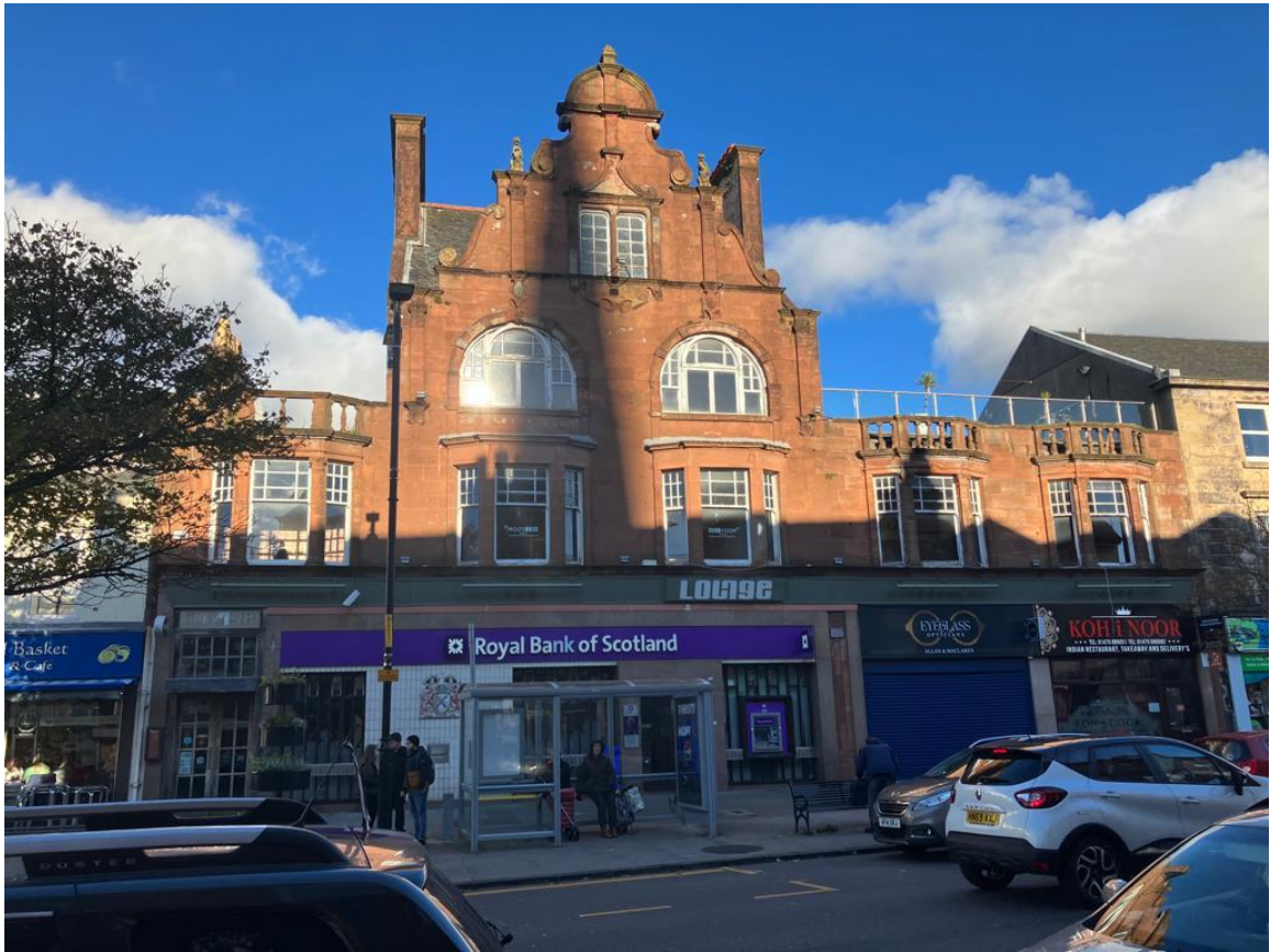
Current Street View Showing First Floor Stone Balustrades And Pinnacles Removed & Ground Level Glazing Dramatically Reduced By Post 1970's Interventions.
