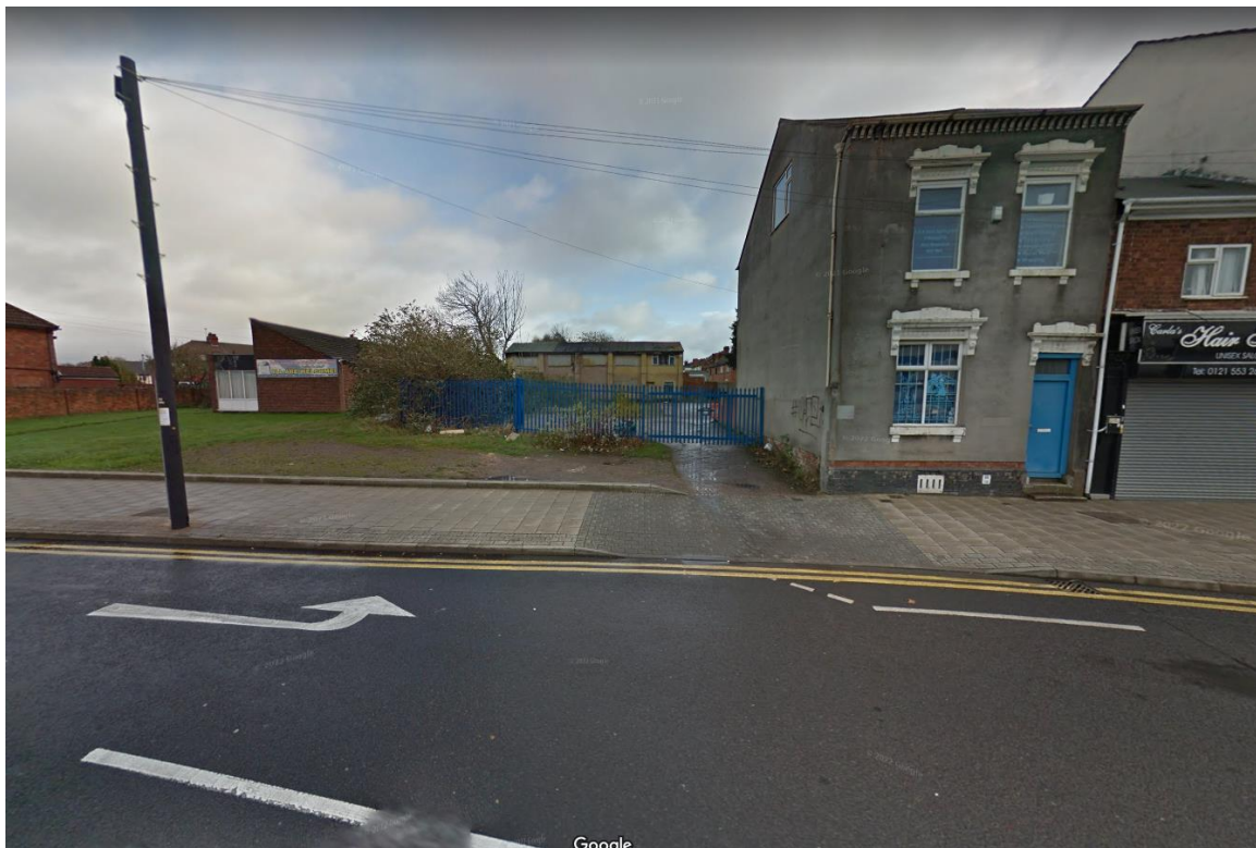
Streetscene view along Walsall Road, leading to Walsall, Bull and Herbert Street intersection.
