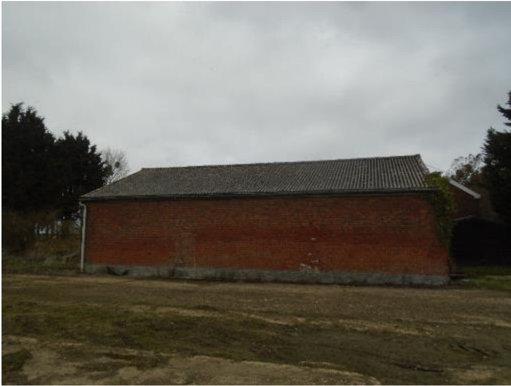
Photo 1. Brickwork on south elevation of the barn.
