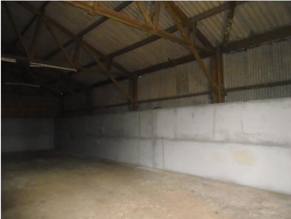
Photo 3. Internal concrete wall.
