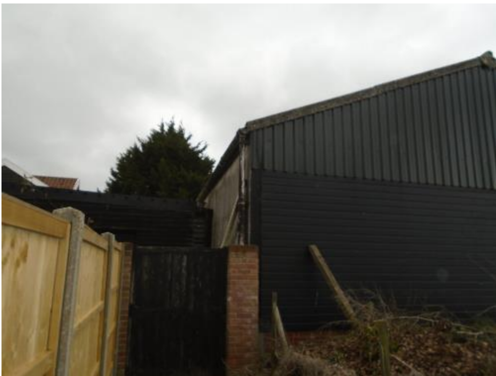
Photo 12. Wooden fence separating the site from neighboring property.
