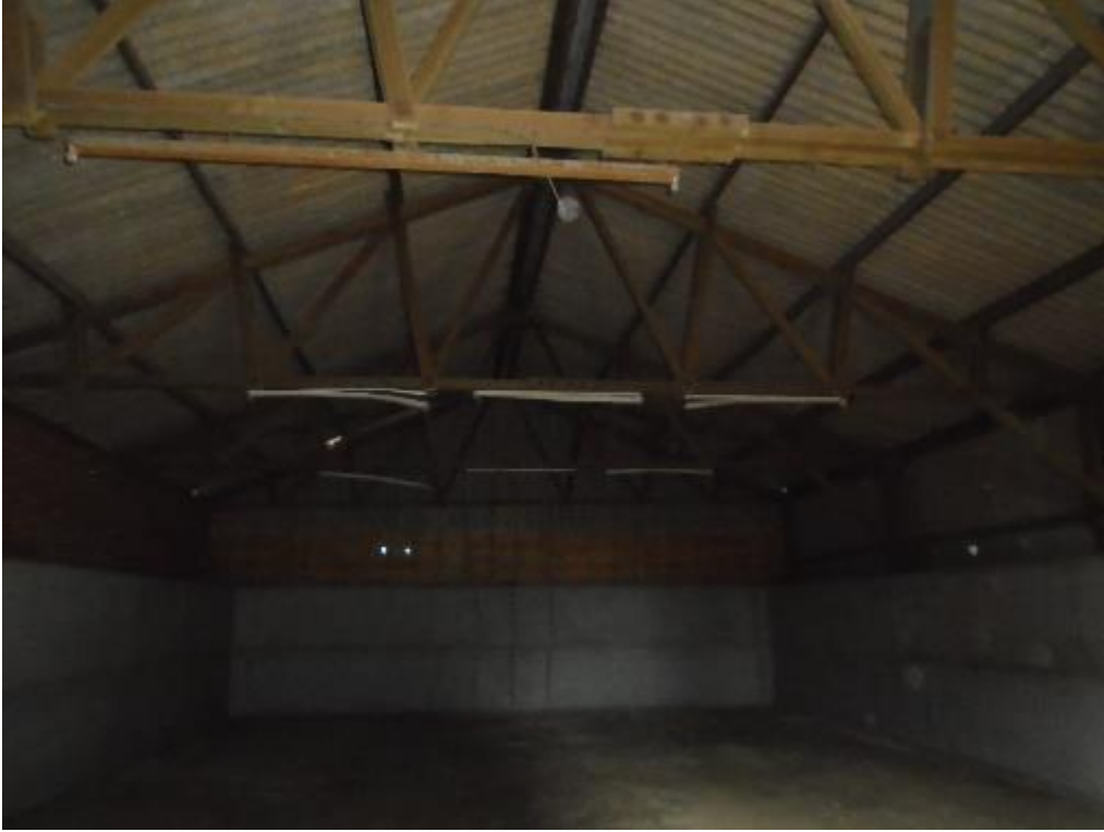
Photo 5. Cement fiber sheeting supported by metal beams.
