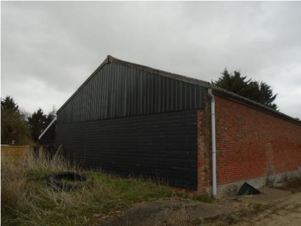
Photo 6. Weatherboard on western elevation.
