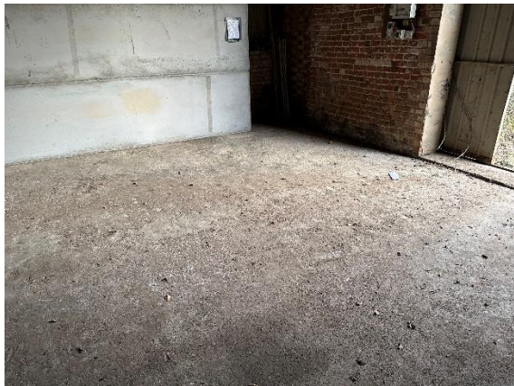
Image 11: Exposed concrete slab internally @ northeast corner
