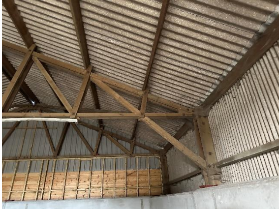
Image 13: Timber braces at truss locations
