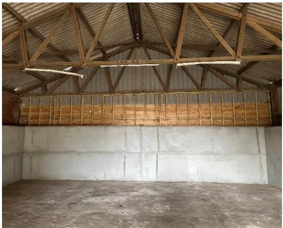
Image 9: Wall Type 2 @ western elevation
