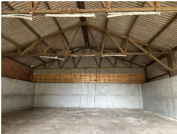
Image 5: View of Existing Timber Roof Trusses
