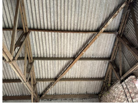
Image 14: Timber diagonal roof bracing
