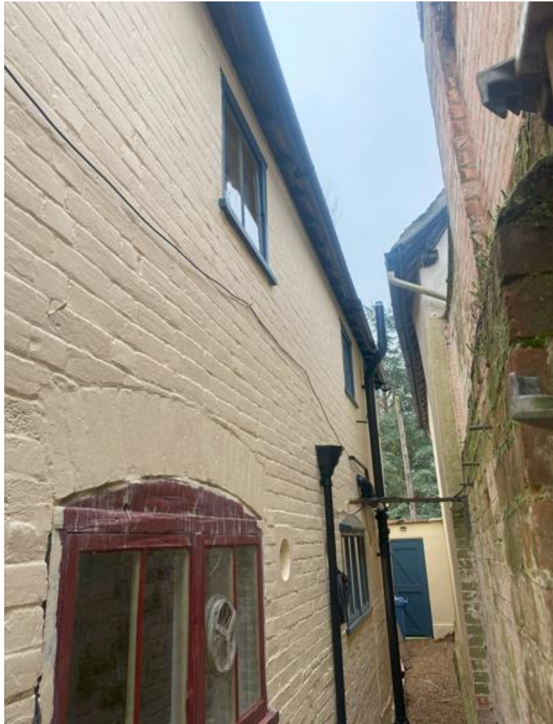
View D From backdoor towards the front gate.
