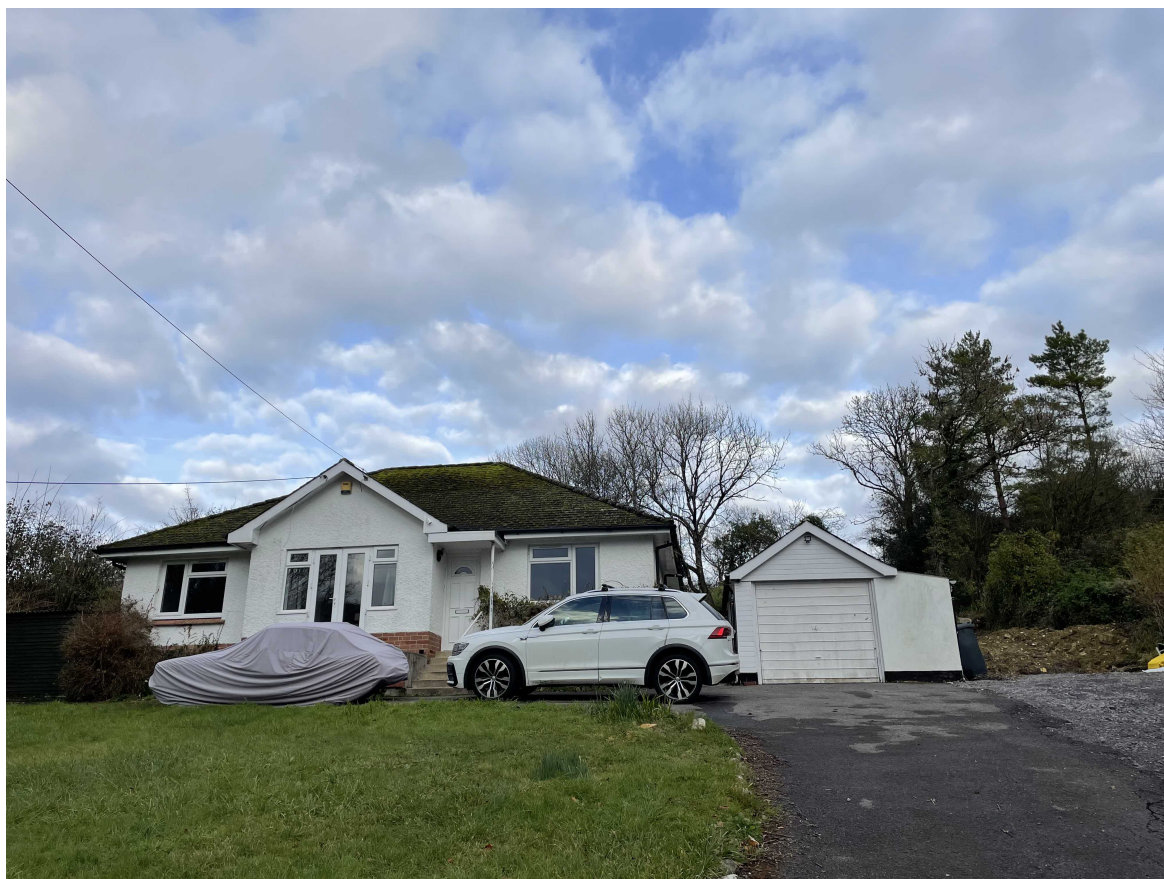
Photograph 1 - Illustrating the existing bungalow 'Nostra Domus'.
