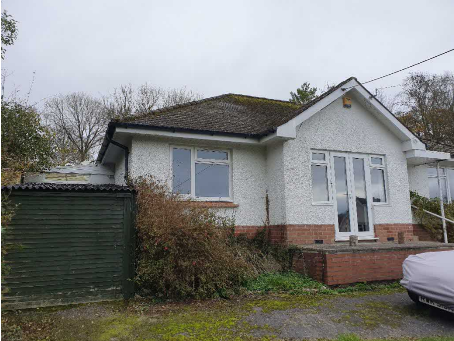
Plate 1 – Southwest facing elevations of the residential dwelling and shed
