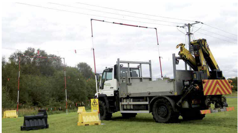
Figure 5 Typical passageway through barriers
