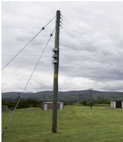
Figure 3 400 V distribution line
