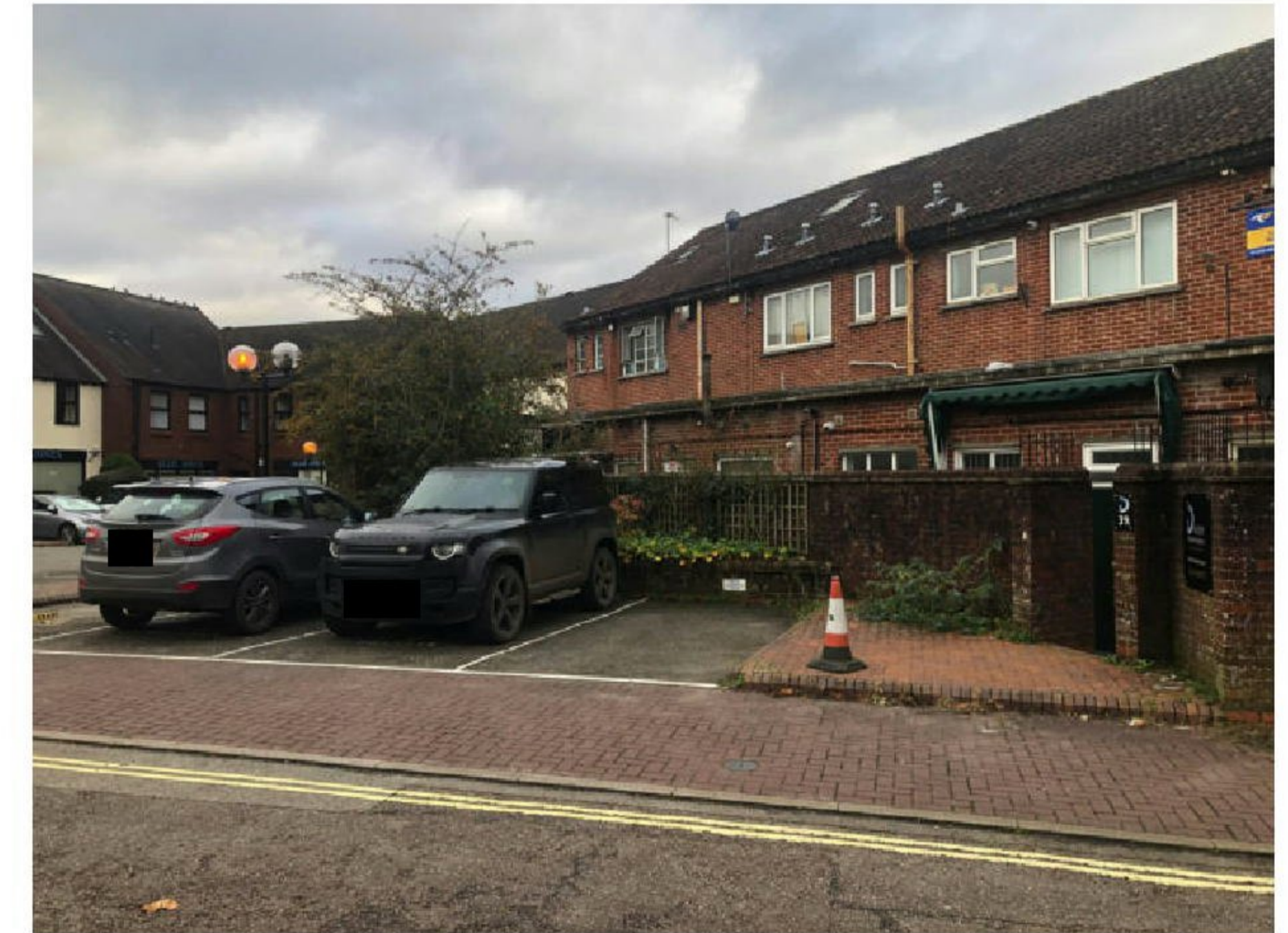
3. View of existing parking to rear of Body Consultancy
