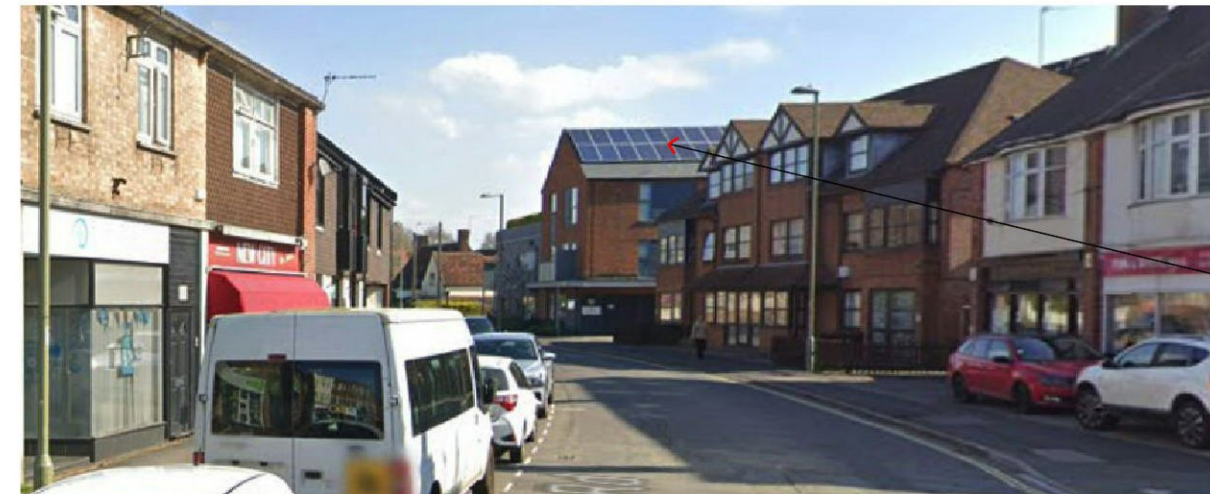
PV panels installed on roof in Southampton Road
