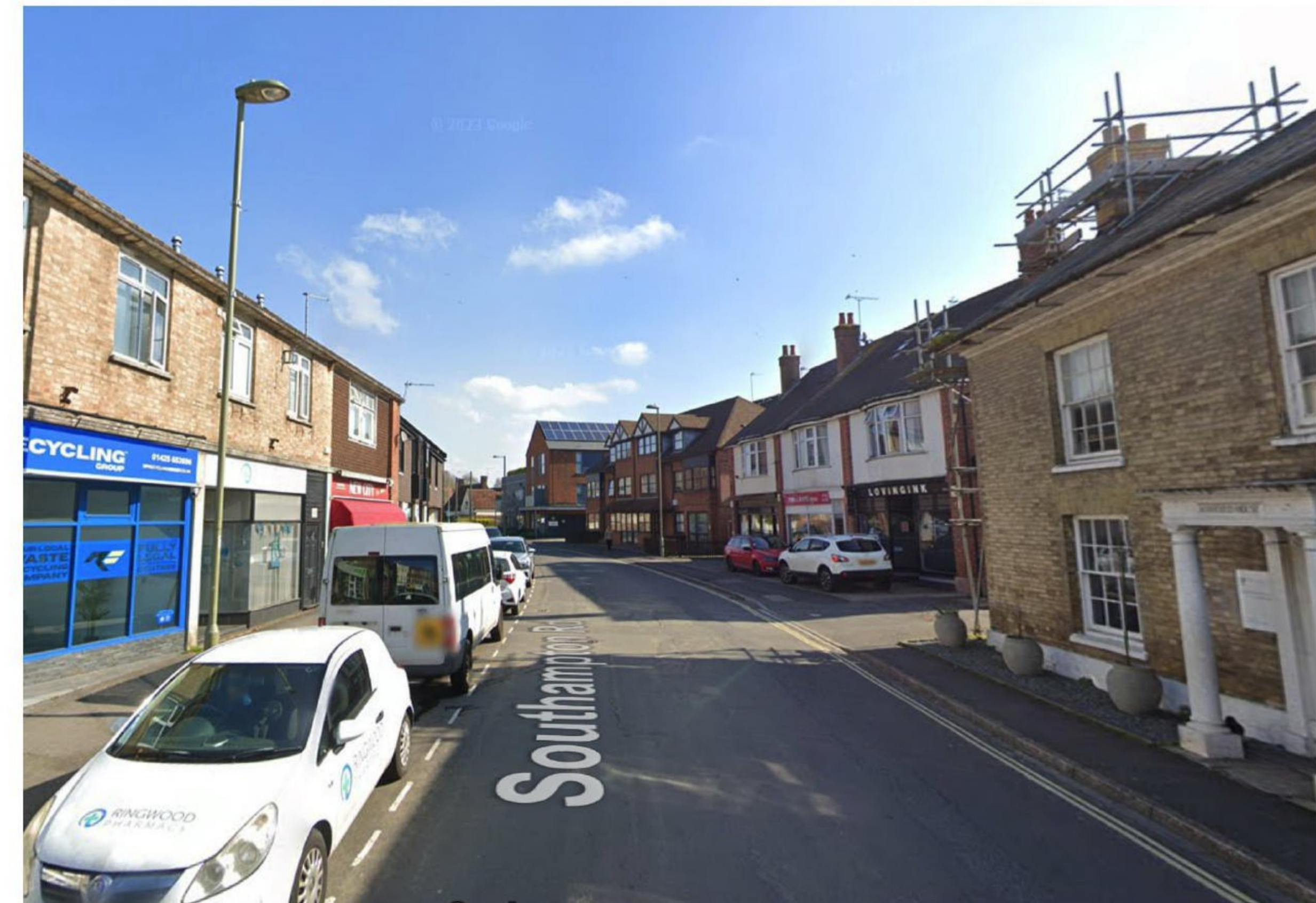
View looking north along southampton Road
