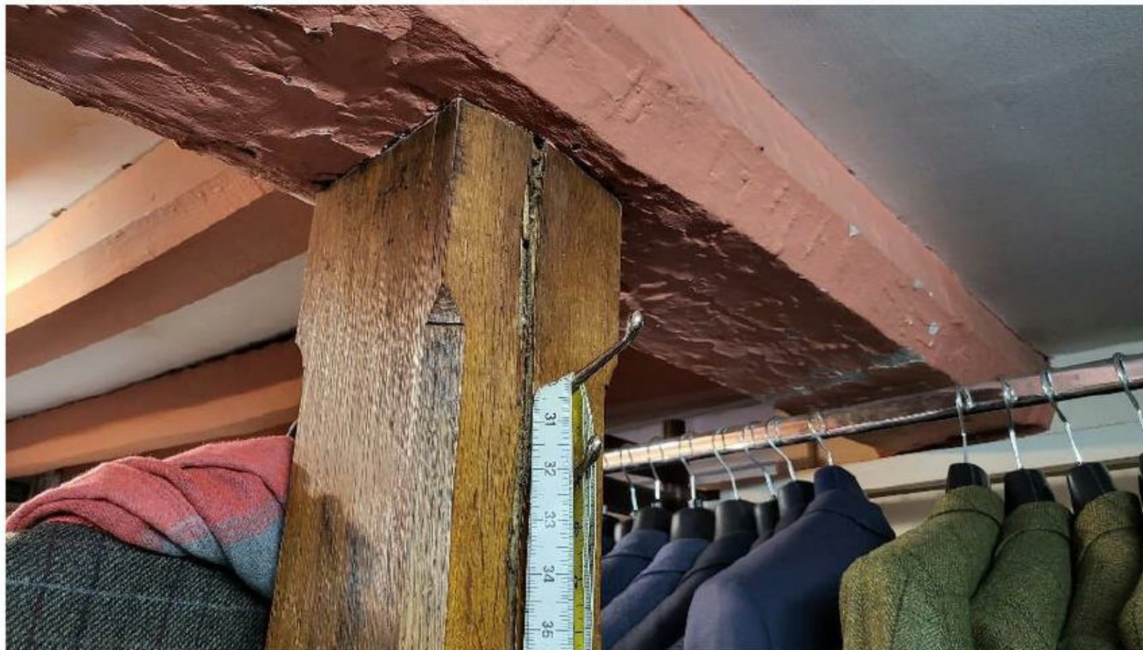
Timber frame behind shop window.
