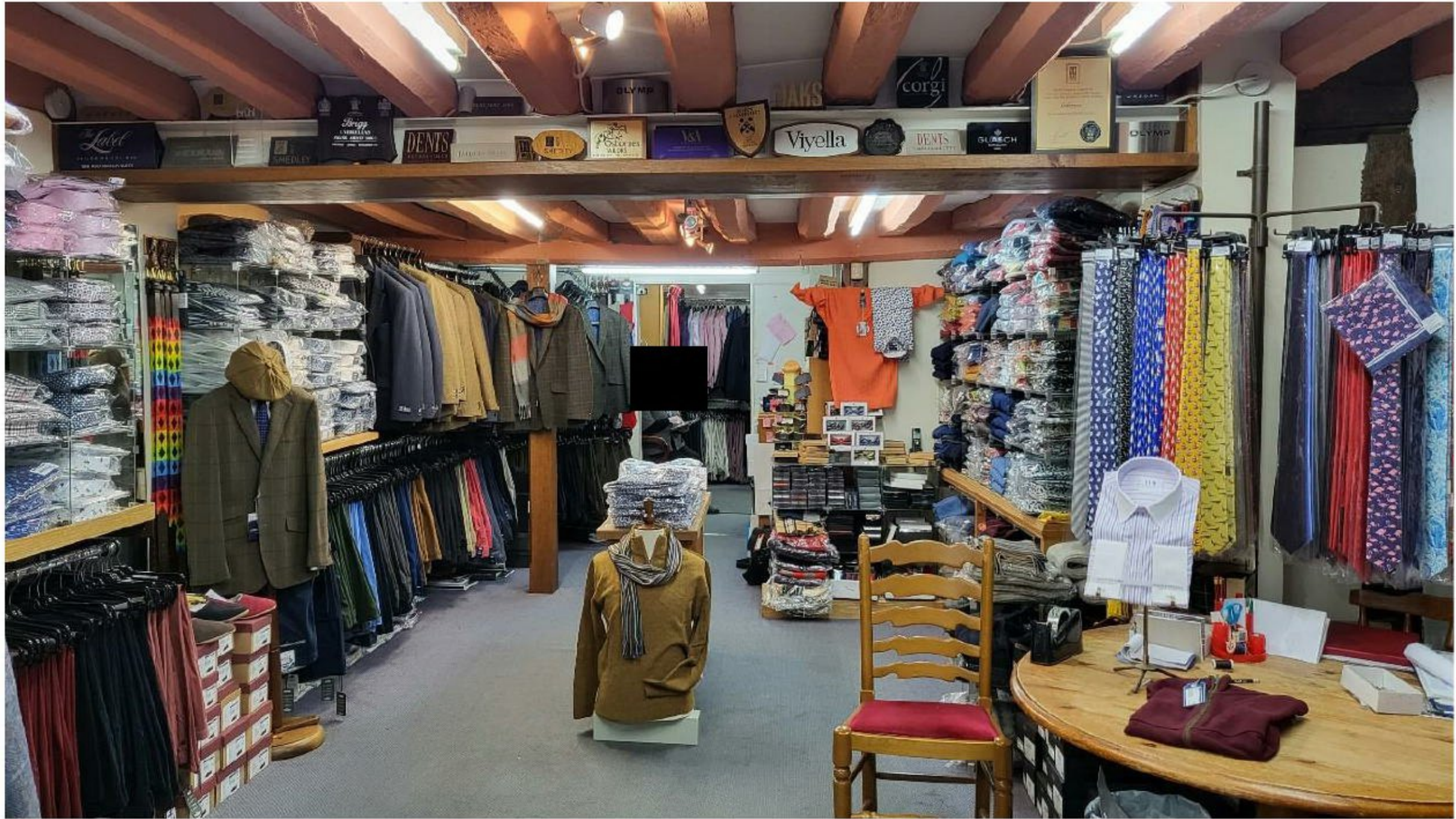
Timber frame running back through shop .
