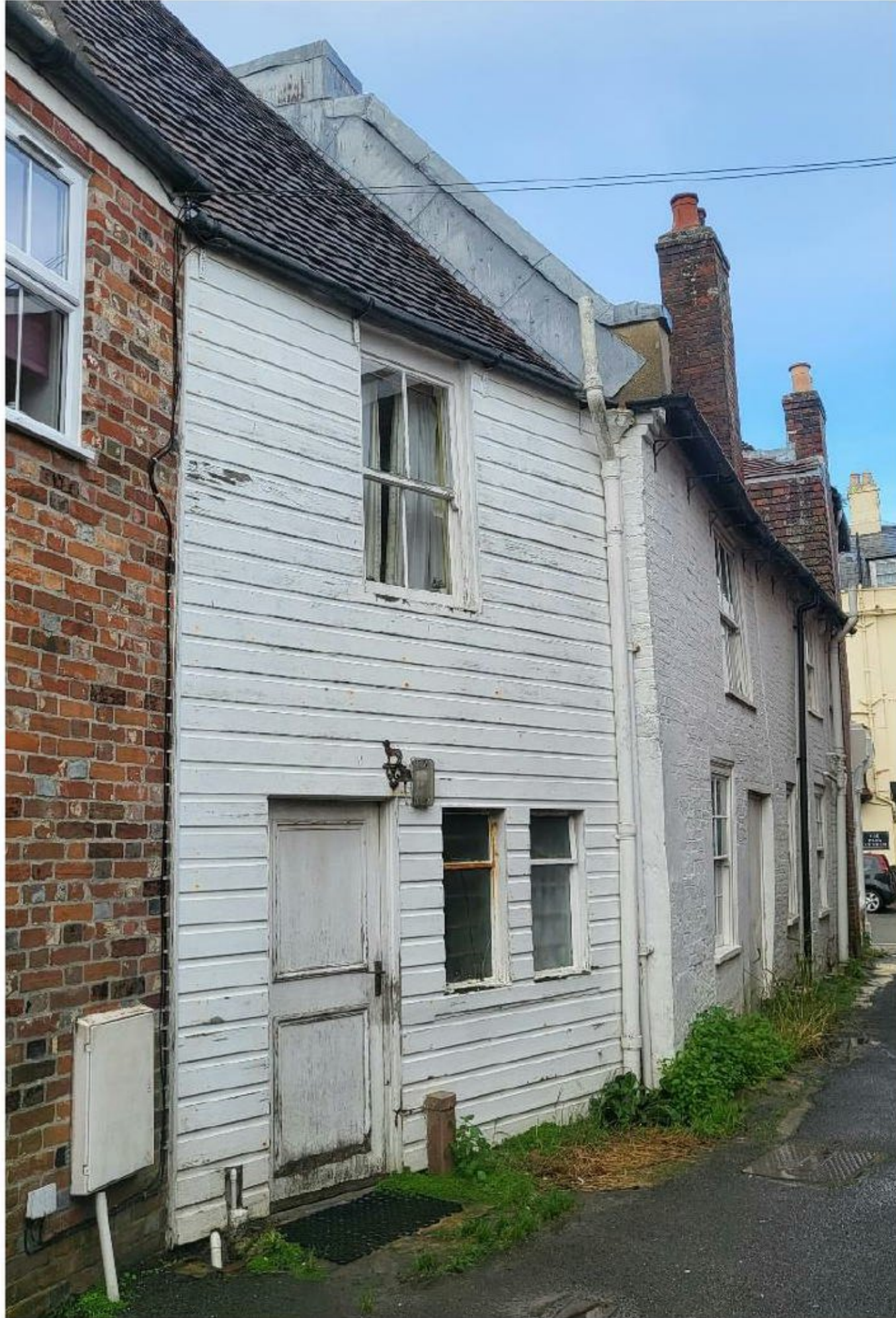
The lead-capped chimney and poor refurbishment of the timber-clad element
