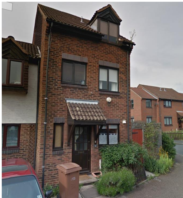
Loc. A – Original South Elevation
