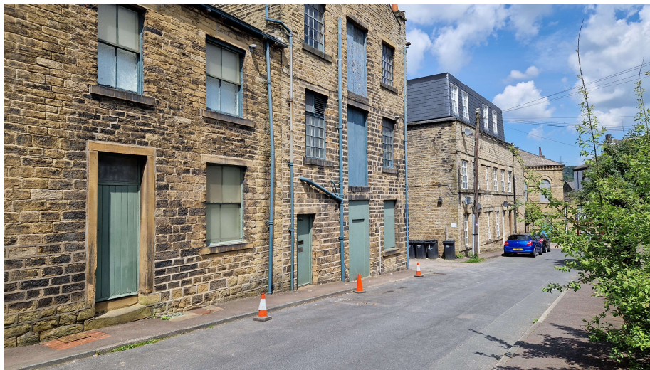
Three storey mill section with existing house to the LHS
