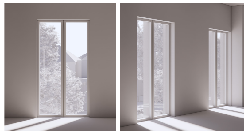
A typical first floor window as viewed internally head-on and then from an oblique angle.
