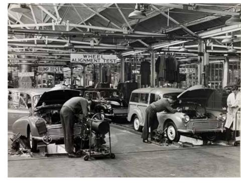
**Figure 4.14** Wheel alignment test, 1959 (source: British Motor Industry Heritage Trust)
