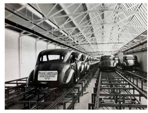
Figure 4.19 Interior of factory building showing roof structure and glazing of sawtooth roofs, 1951 (source: British Motor Industry Heritage Trust)
