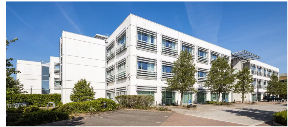
Figure 10. Oxfam House, John Smith Drive
