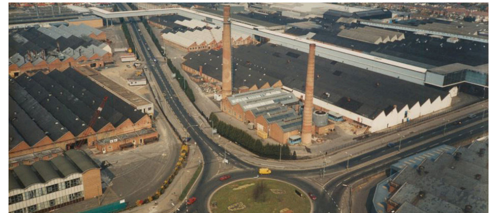
Figure 13. Historic Photo Of Cowley Roundabout
