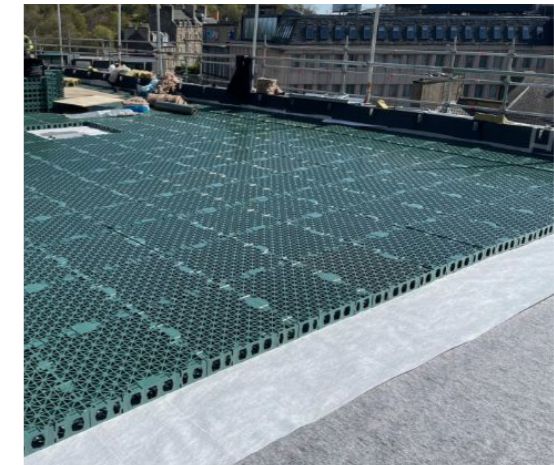
Figure 42. Blue roof system
