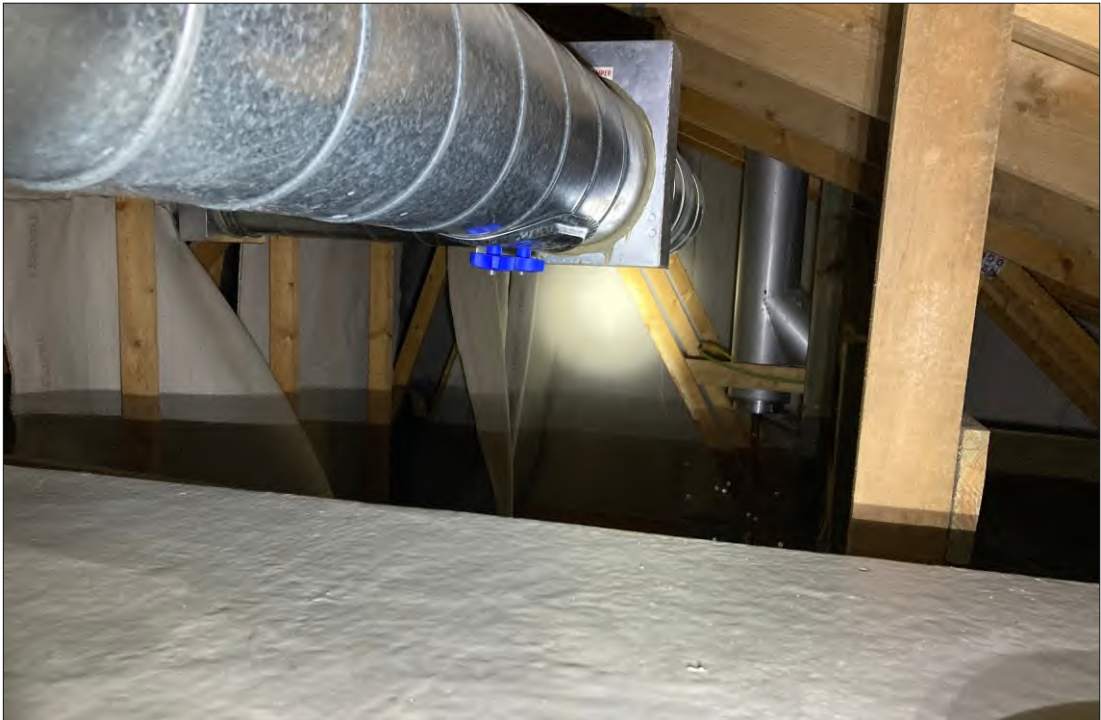
PHOTOGRAPH 6: Loft Void within Building
