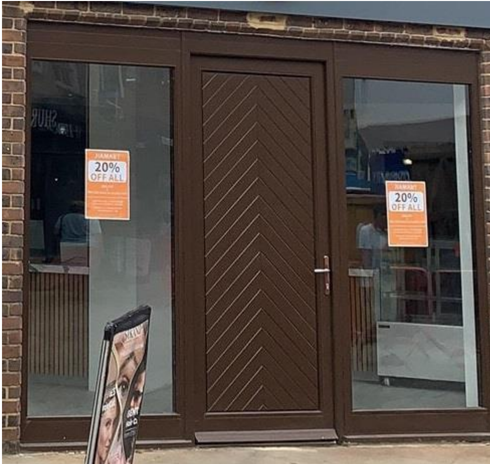
DOOR ON SOUTHWEST ELEVATION
