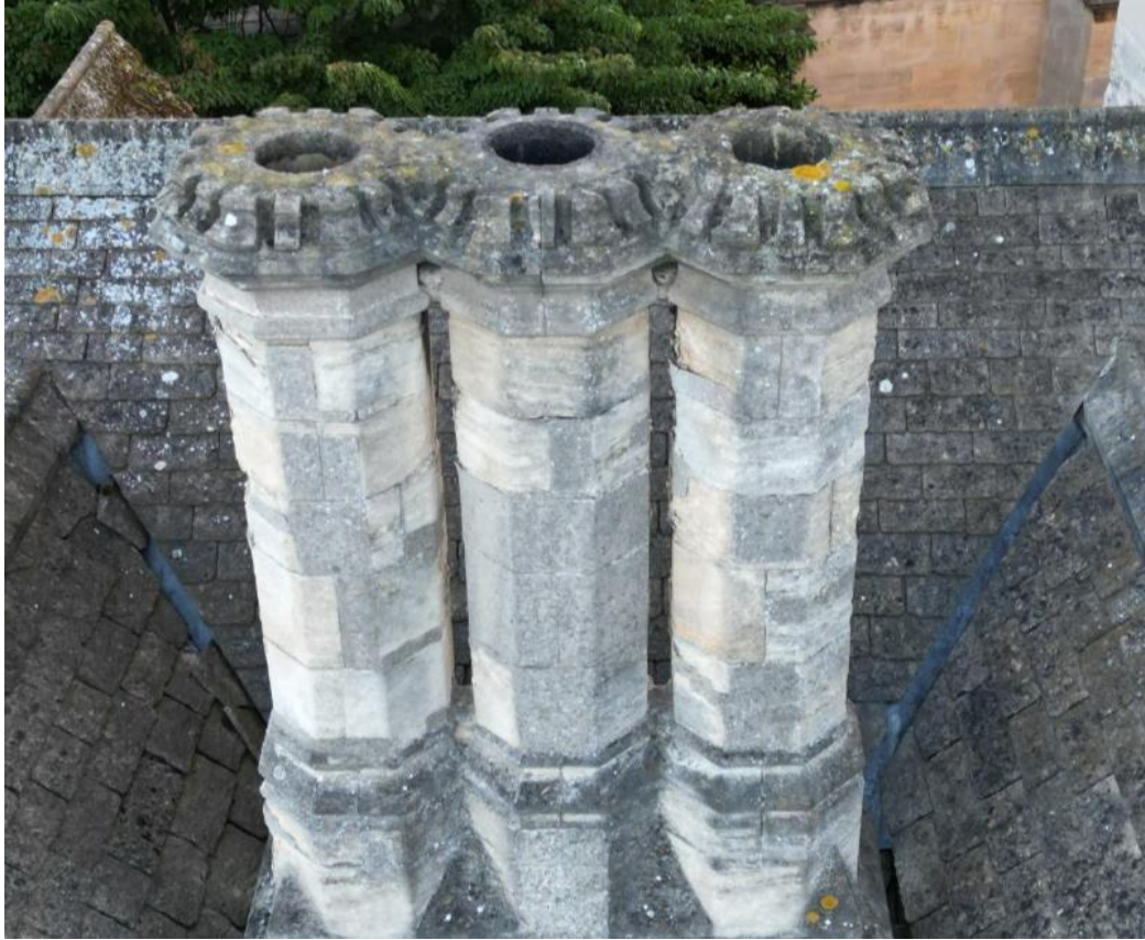
Fig. 3 Chimney stacks – High Street elevation
