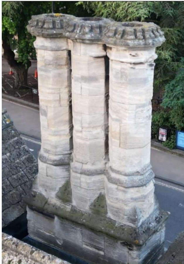
Fig.7 Chimney stacks seen from the north
