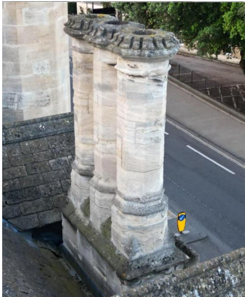
Fig.6 Chimney stacks seen from the west
