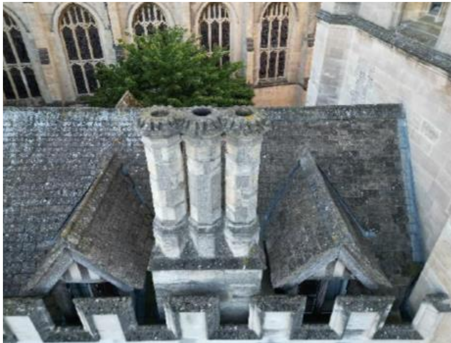
Fig. 2 Chimney stacks High Street elevation
