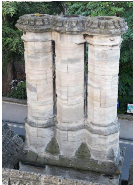
Fig 9. Chimney stacks seen from the north
