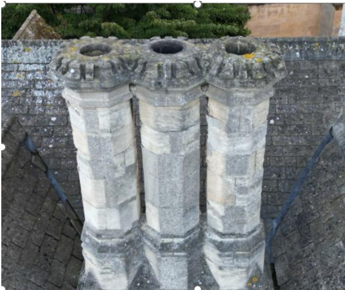
Fig 2. Chimney stacks – High Street elevation
