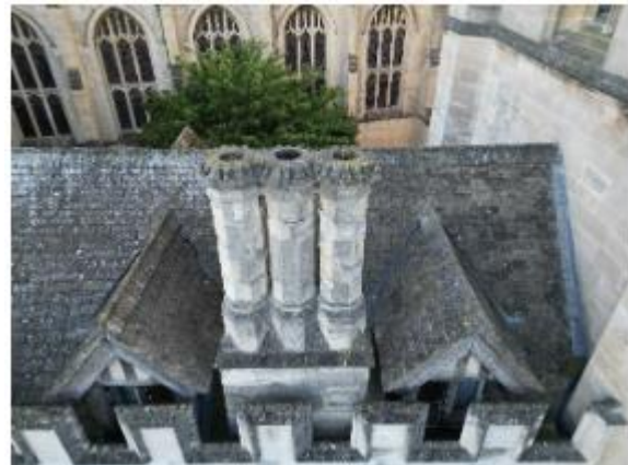
Fig 1. Chimney stacks immediately to the west of the Great Tower
