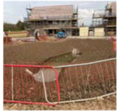
Attenuation Pond Viewed from south
