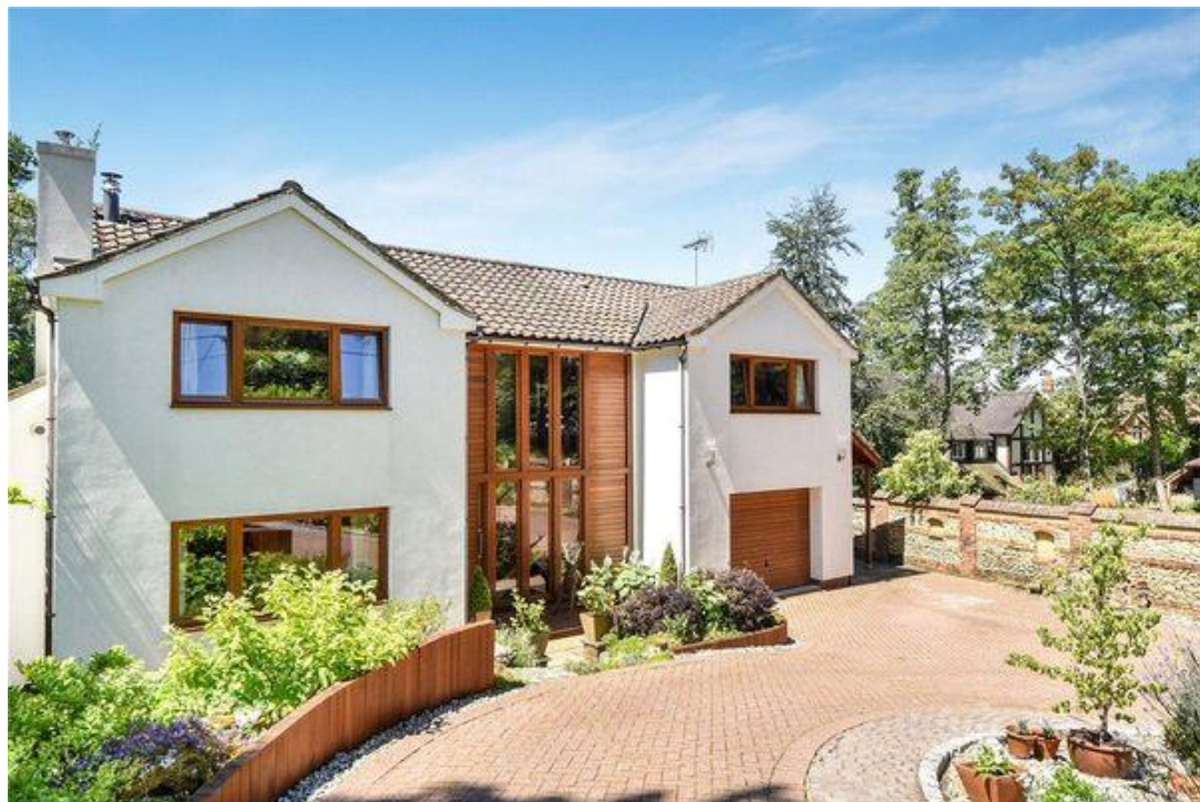
Fig. 3 – Photograph of the existing east elevation taken from the driveway
