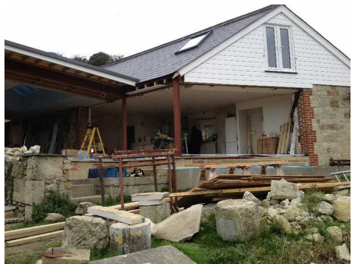
View of alterations to the rear of property in progress
