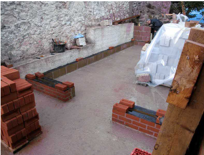
View of western extension under construction
