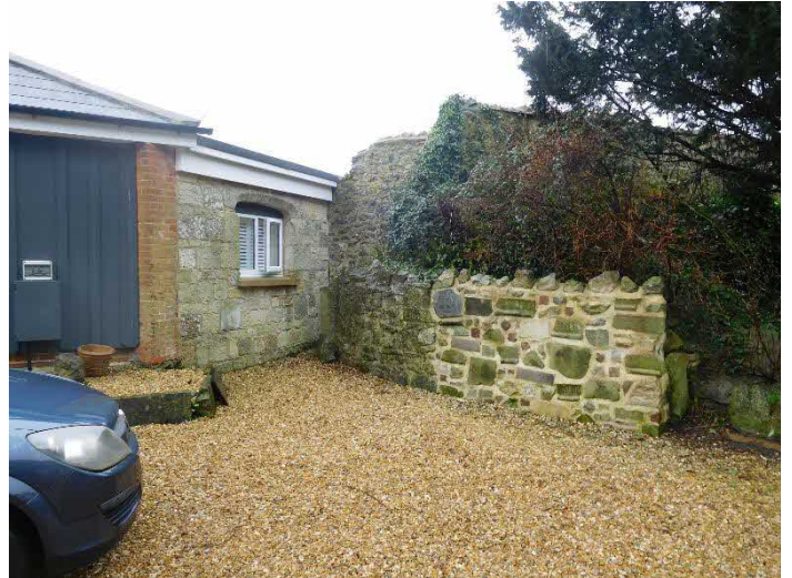
View of western side extension and historic stonewall
