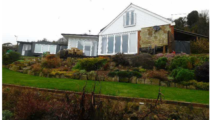
View of rear elevation from lower garden terrace
