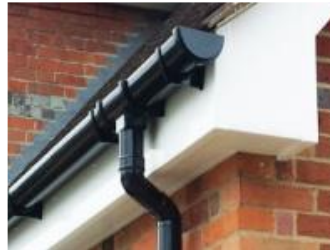
Gutters & Downpipes - Black UPVC
