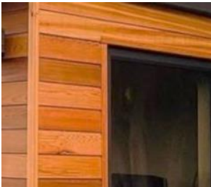
Weatherboarding – Western Red Cedar
