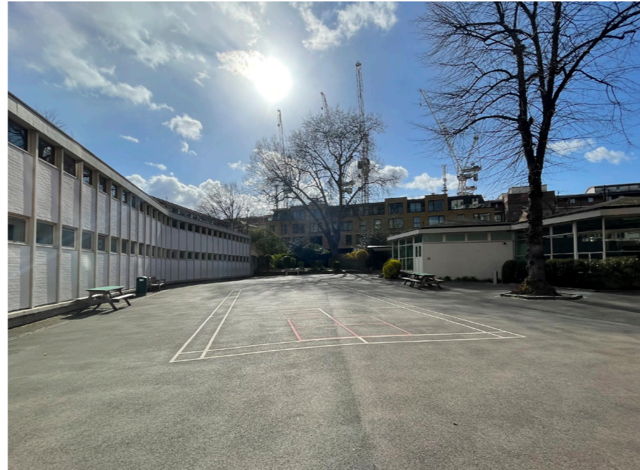
Existing conditions of external area
