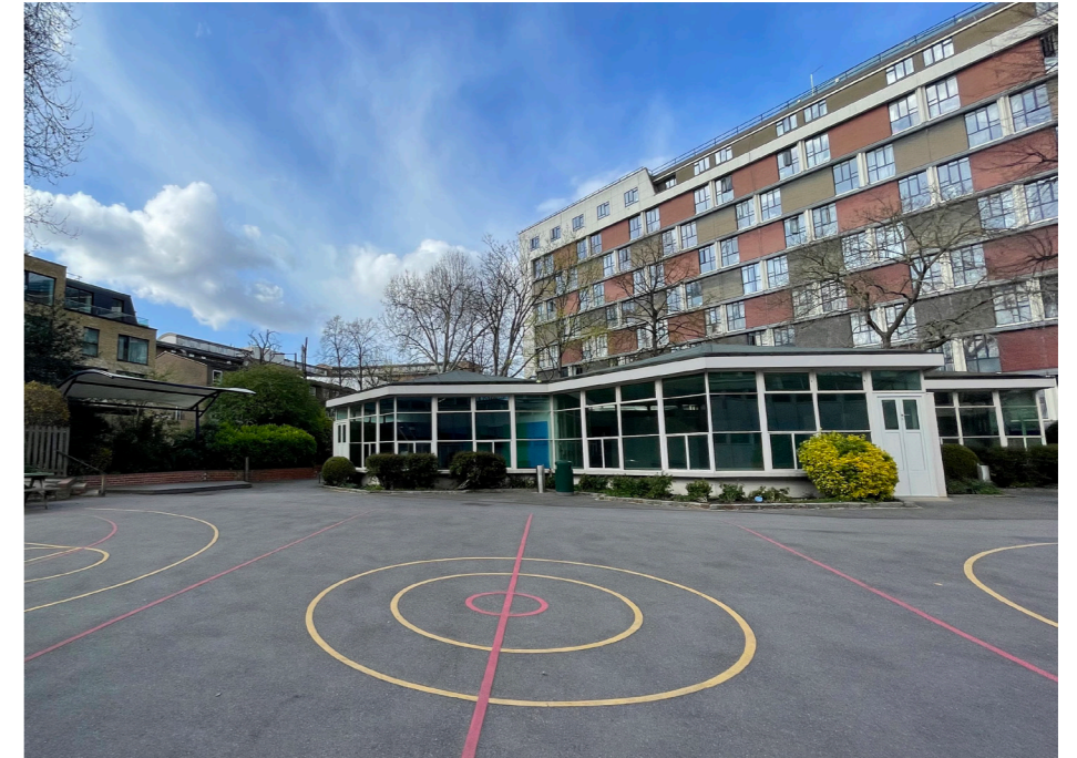
Existing College Park Satellite School building
