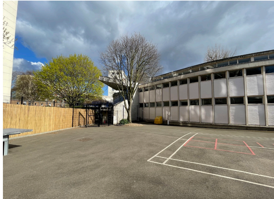
View towards main School Building showing existing fencing
