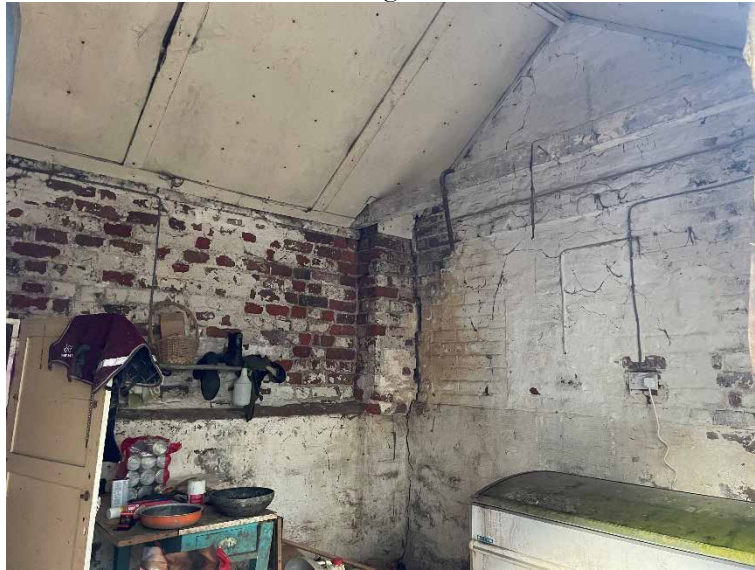
Plate 9 – Outbuilding, internal roof void.
