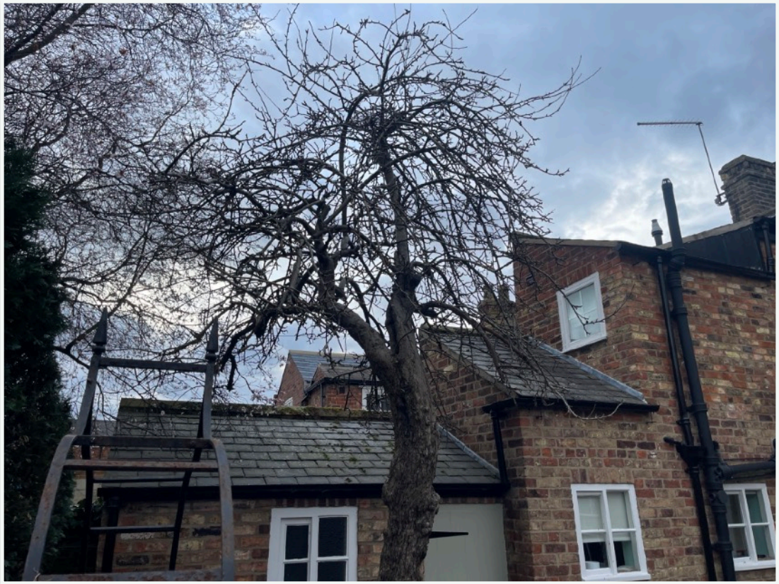
Figure 3. T1 with a canopy biased over the neighbouring building.
