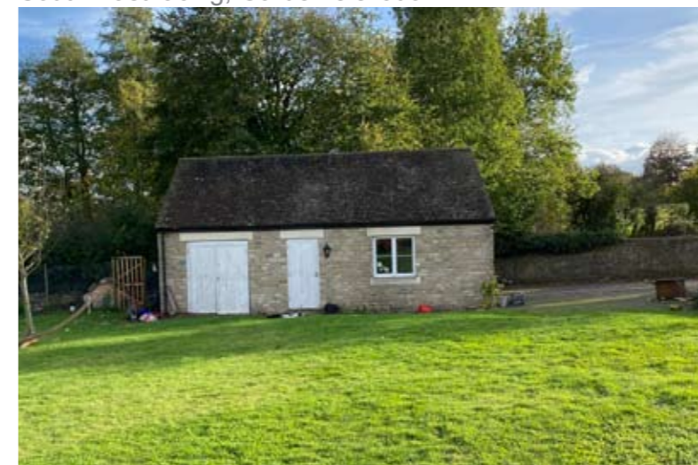
Garage - North facade
