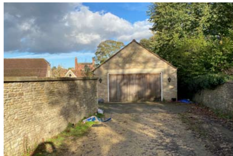
West facade view of 2010 garage from rear driveway
