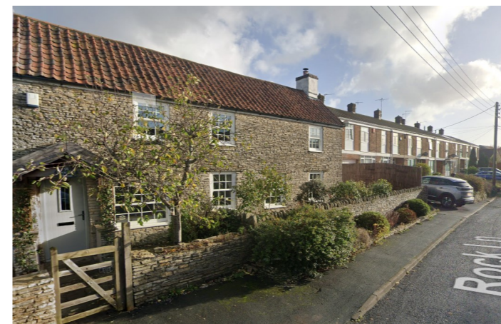
The stone wall and boundary wall of no.96 Rock Lane
