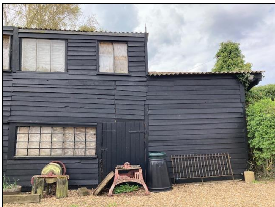
Plate 7: North-east elevation, north end
