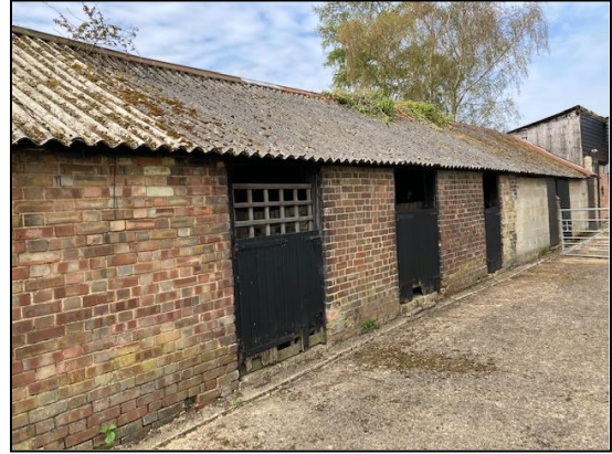
Plate 2: North-east elevation looking north
