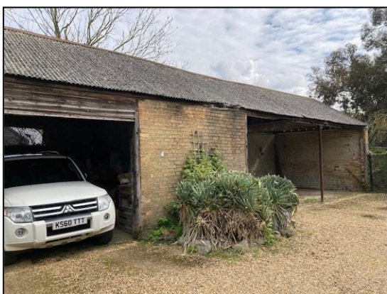
Plate 15: Southern elevation, north end
