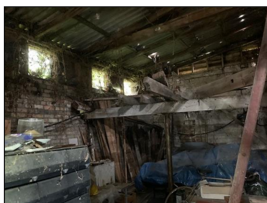
Plate 12: Interior, north-west corner
