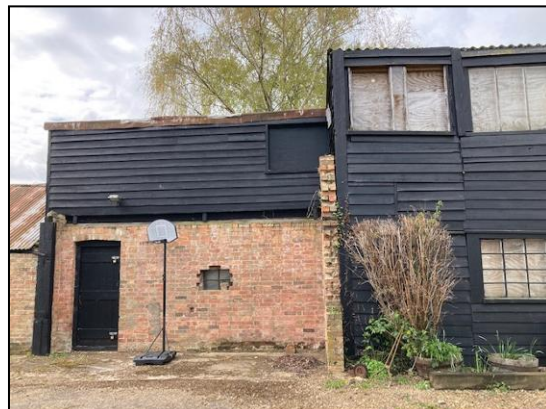
Plate 8: North-east elevation, south end
