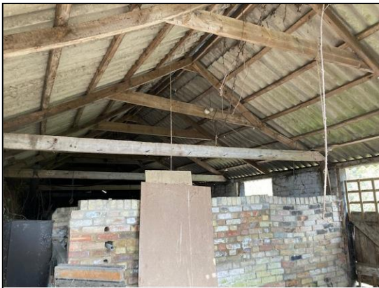
Plate 3: Interior, south end
