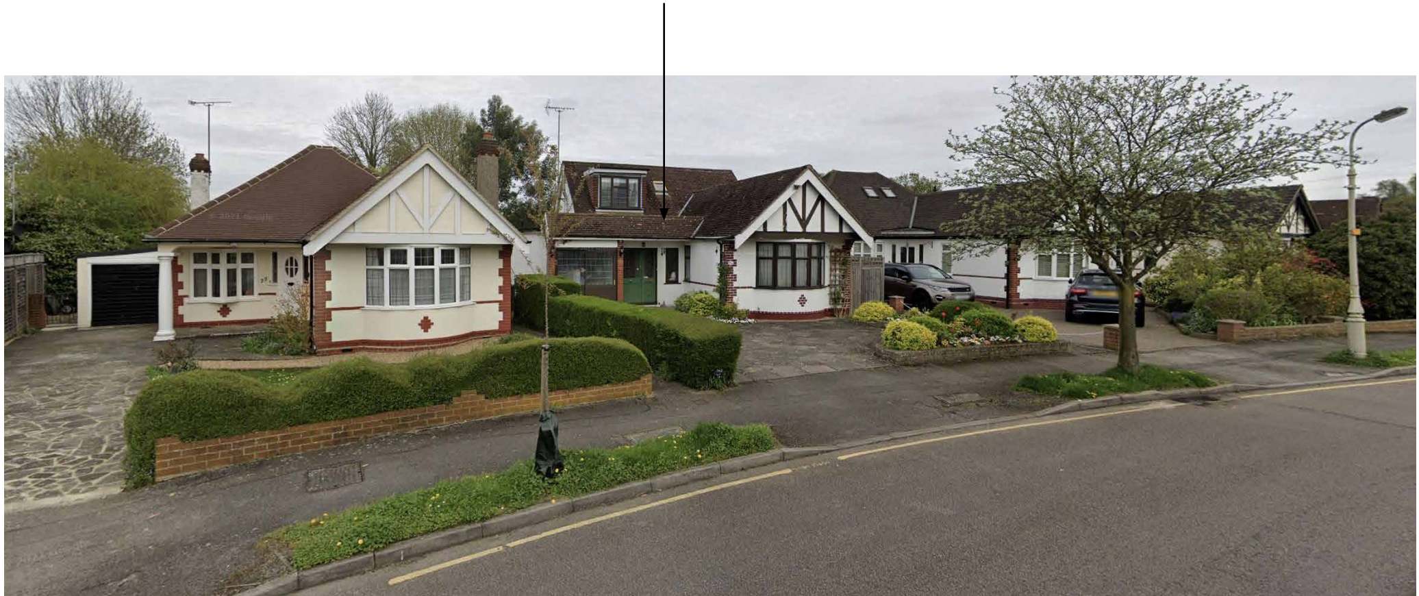
24 Elmroyd Ave, extended with a hip to gable extension and side infil Garage
