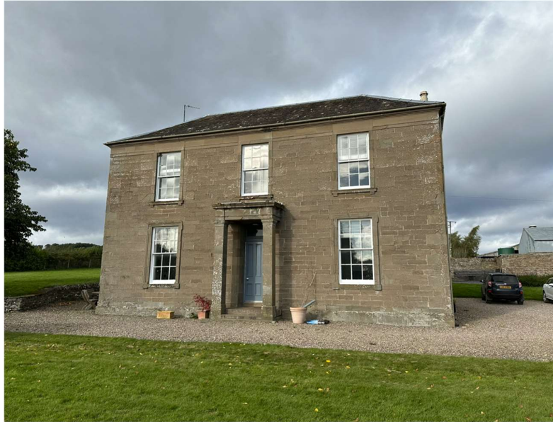
Figure 1 - Photograph of south elevation showing existing primary access point to dwelling.
