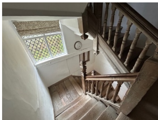
Stair viewed from 2 nd floor.
