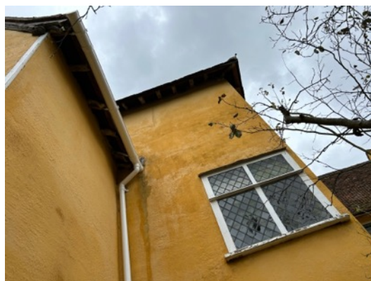
WG1 and gutter overflow above.
