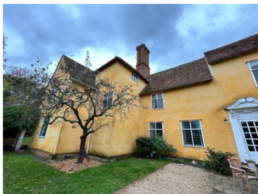
Stair tower viewed from south east
