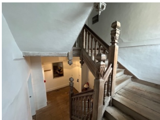
Stair viewed from ground floor half landing
