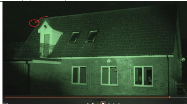
A bat recorded flying low over the ridge of the building during the first survey (21/06/23). This is a view of the north elevation.
