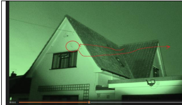
Emergence from under the roof tile on southeast gable (21/06/23).
