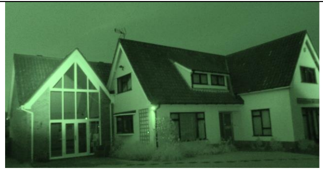
Infra-red camera view from the 21/06/23 of the south elevation and western extension and gable ends.
