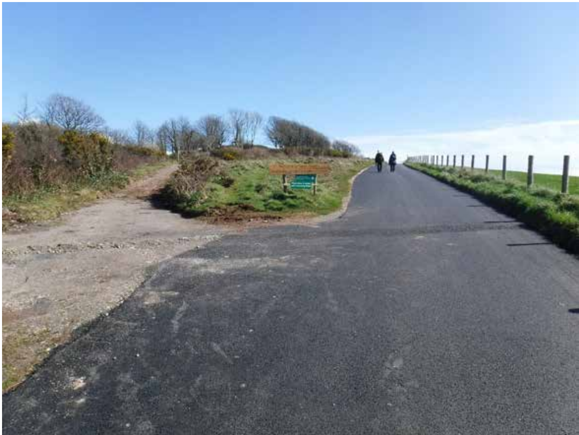
Fig 14 The entrance to Maker Heights. The recently resurfaced Tarmac road on the right will be the route in and the hardcore track on the left the exit.
