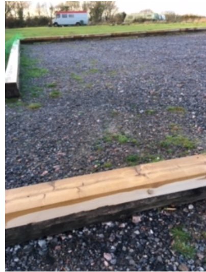
Figure 11 Main Car Park following resurfacing
