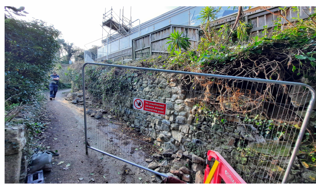
Figure 2: Photograph showing East elevation.
