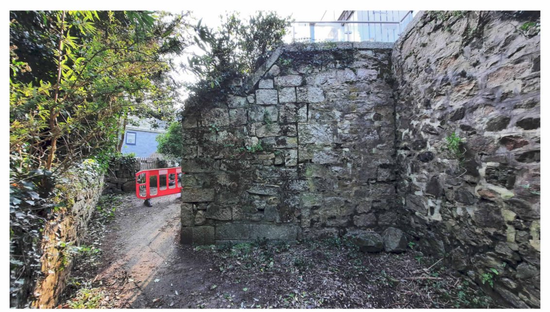
Figure 1: Photograph showing North elevation.
