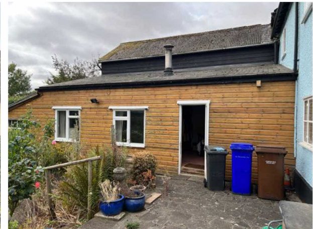
Principal North Elevation (rear wing/side)
