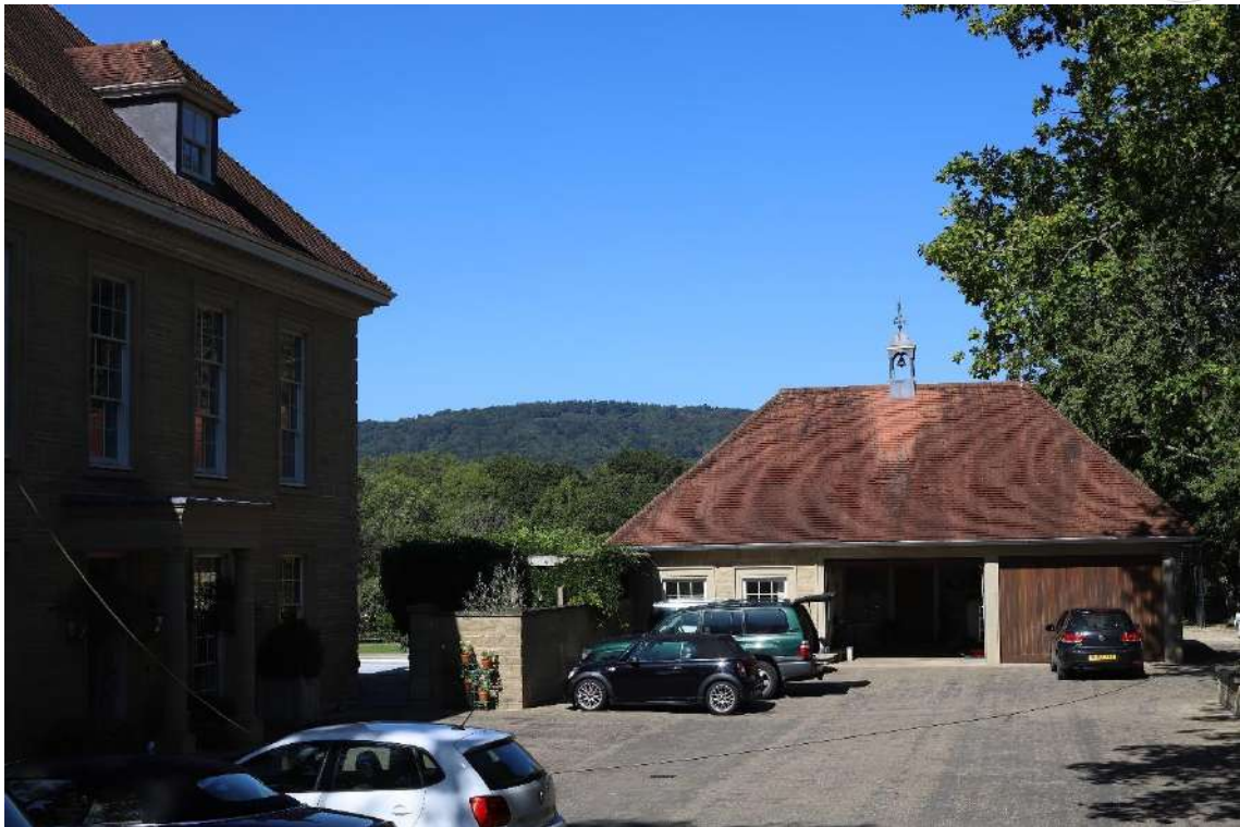
Plate 2 View of the existing garage.
