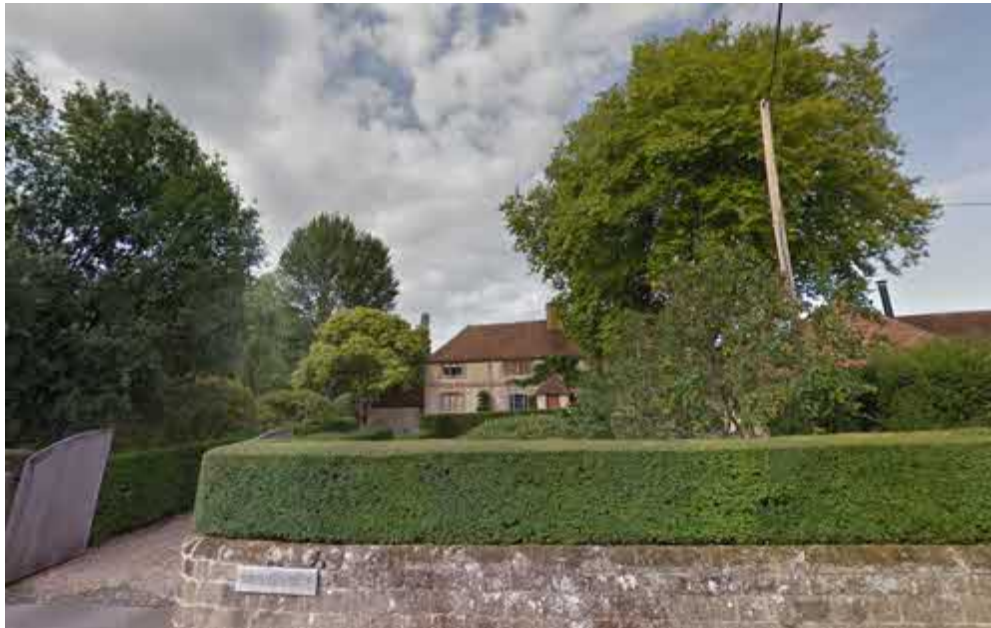
The east elevation of Bridgefoot. ©Google
