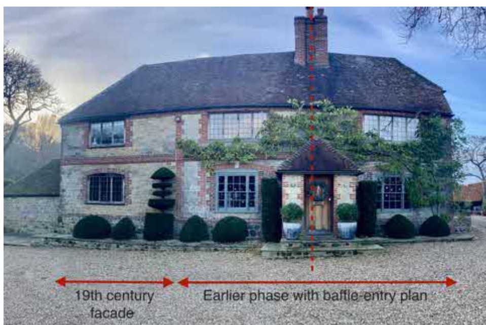
The façade of Bridgefoot showing the two phases with the earlier phase to the north.
