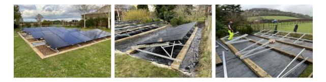
No concrete or aggregate will be used in the construction, and no base is required. There is no requirement to bring soil in or out of the site area for construction.
